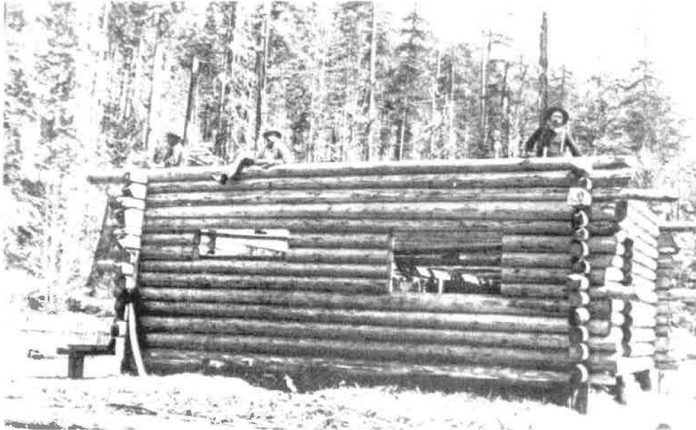
Construction photograph, c. 1907 - looking northeast on west façade, USFS Olympic NF Collection
