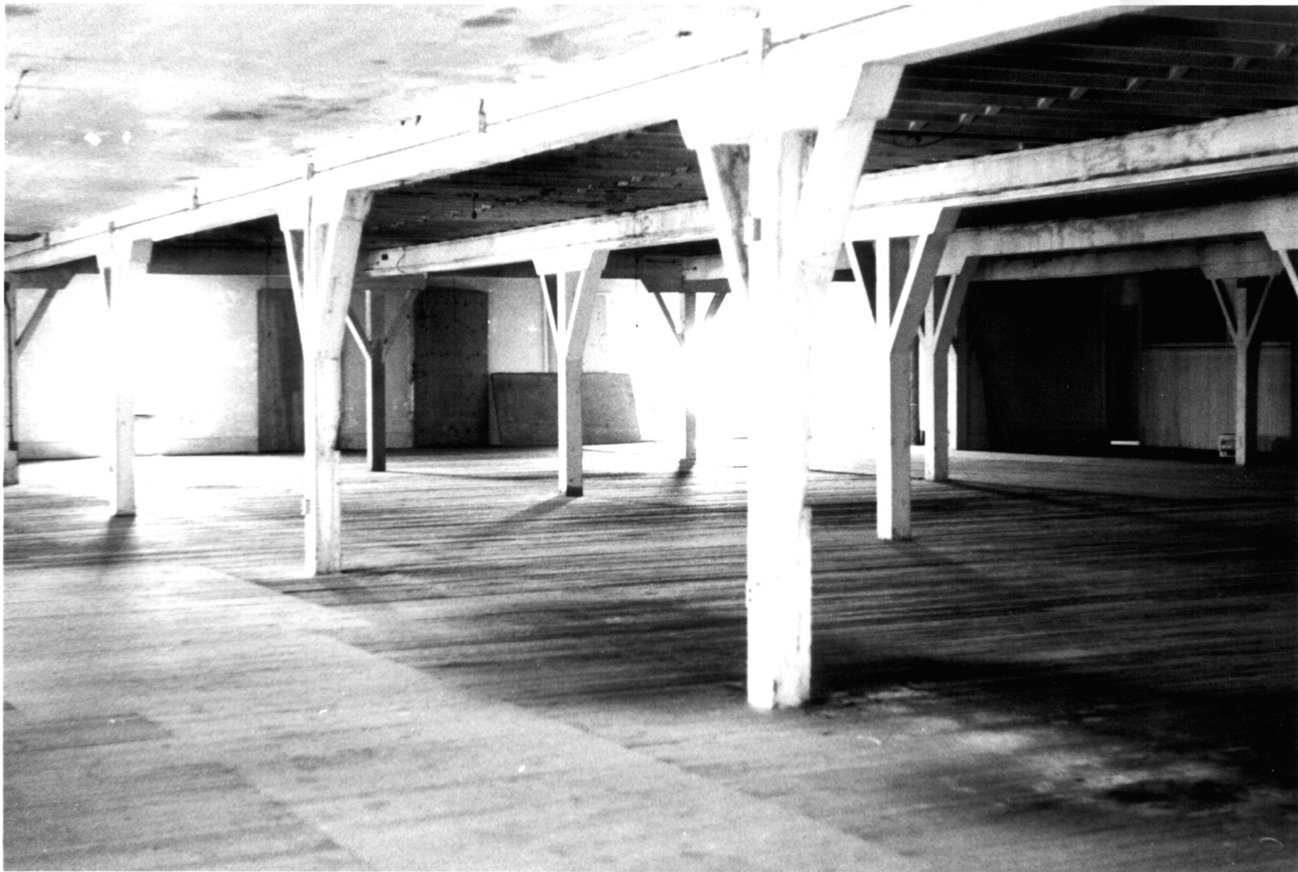
Clay Building, second floor
