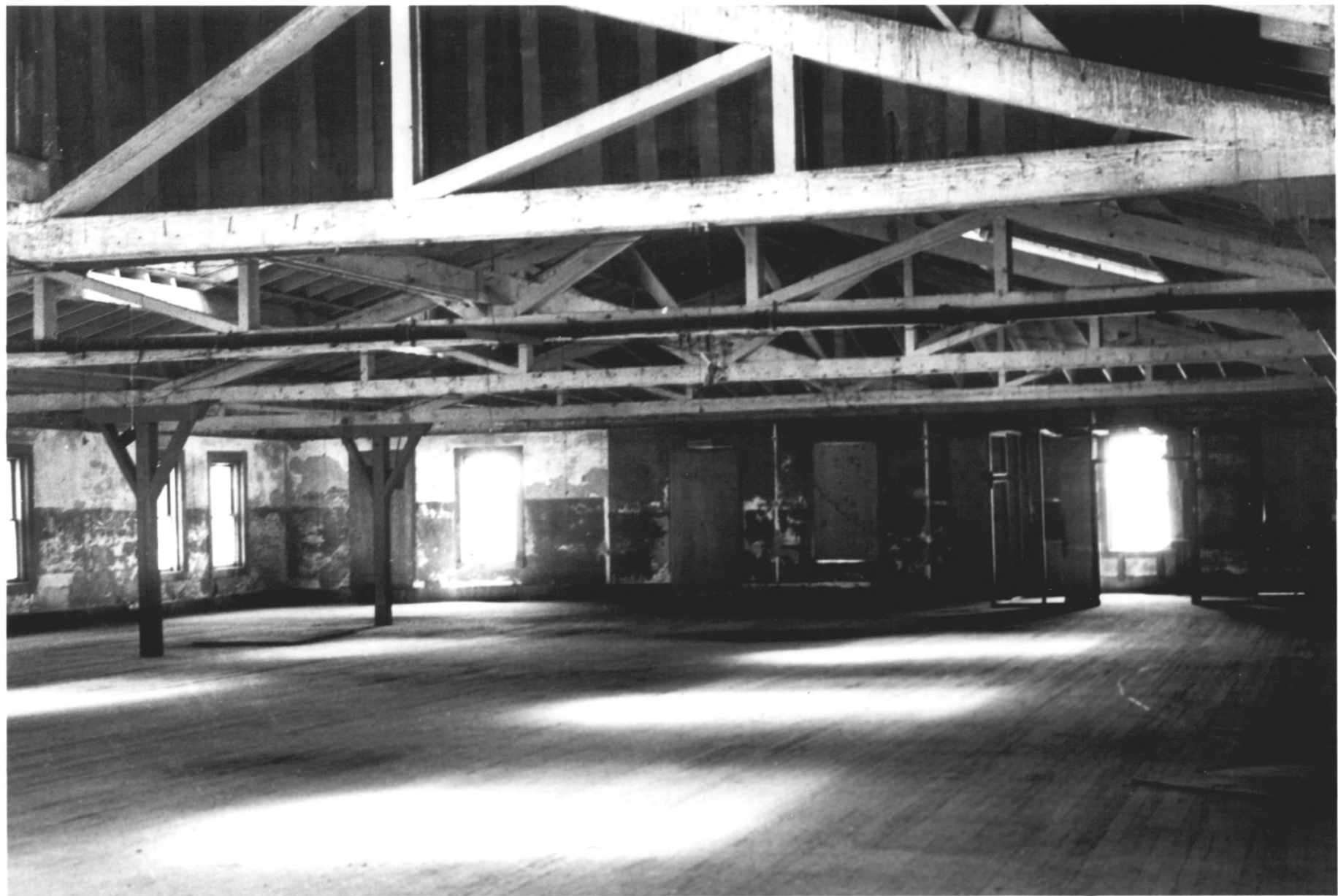
Clay Building, third floor
