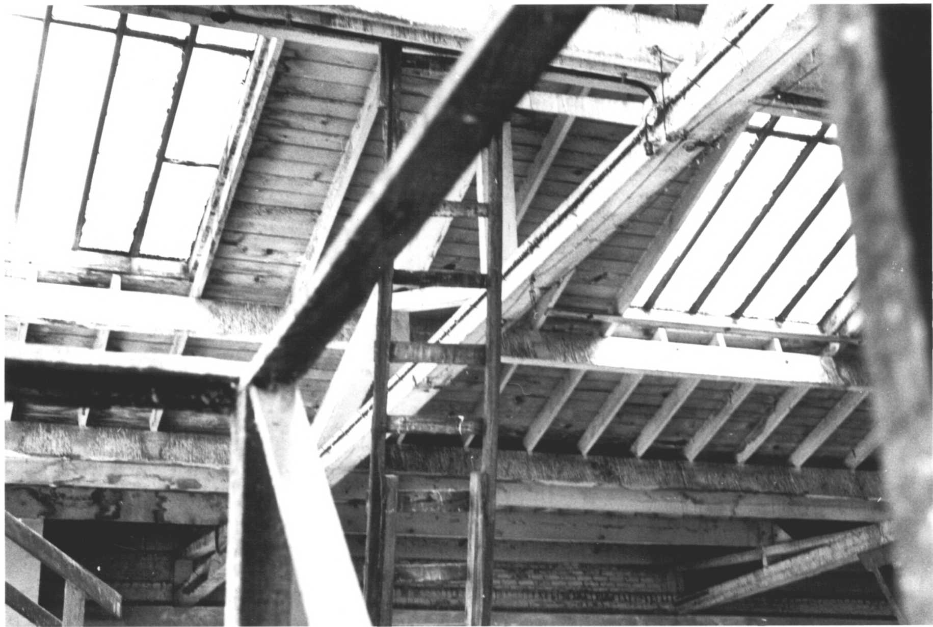
Clay Building, skylights
