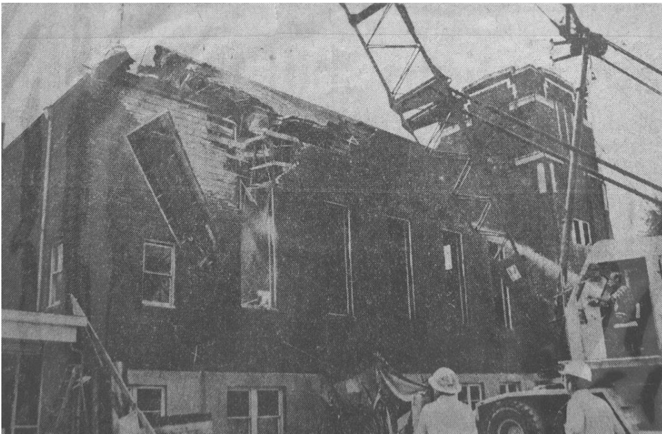
Demolition begins of 1920 church for new sanctuary. Seattle Times : August 14, 1974
