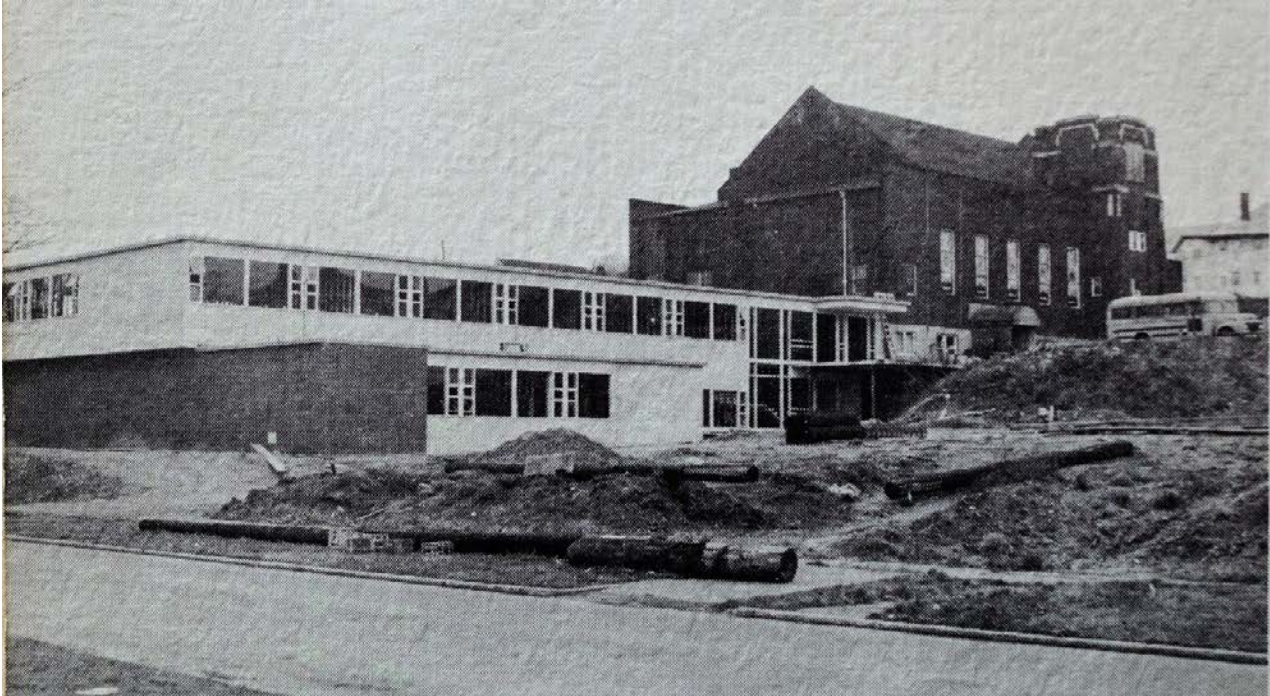
Nearly completed 1963 educational and administrative wing of Mount Zion Church behind 1920 sanctuary. Photo courtesy of http://centralareacomm.blogspot.com/
