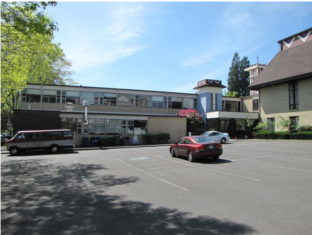
5 of 20 Mt. Zion Baptist Church 1963 educational wing, north facade.
