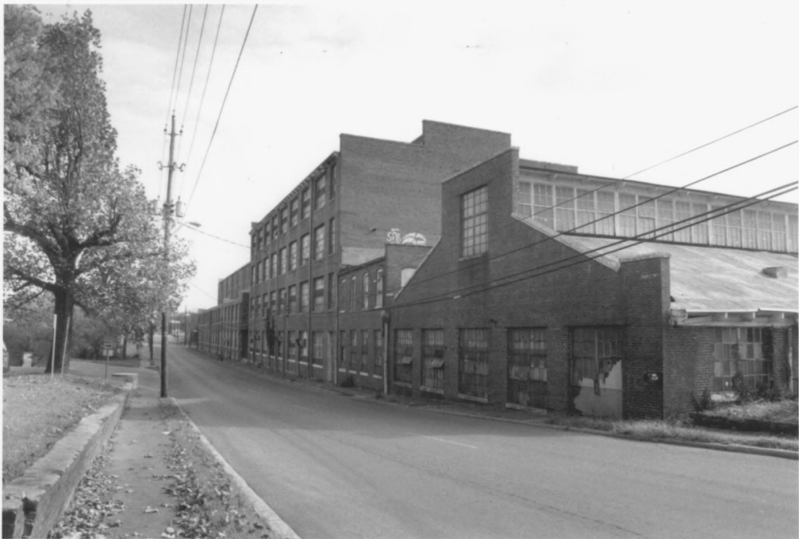
HARDVICK WOOLEN MILLS BRADLEY COUNTY, TN
