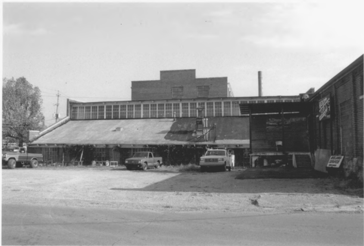
HARDVICK WOOLEN MILLS BRADLEY COUNTY, TN
