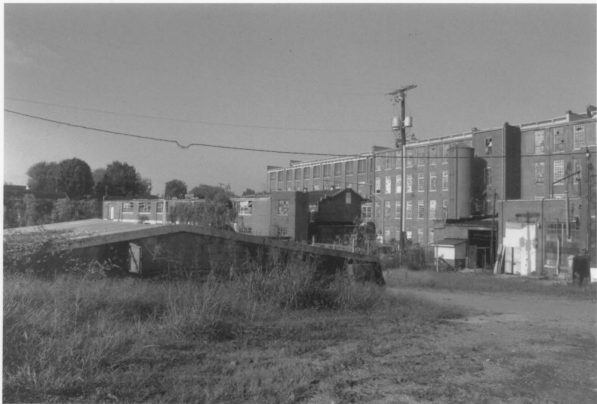
HARDWICK WOOLLEN MILLS BRADLEY COUNTY, TN
