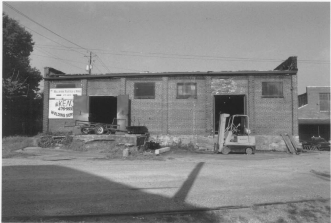
HARDWICK WOOLLEN MILLS BRADLEY COUNTY, TN
