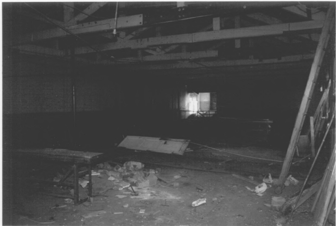
HARDWICK WOOLLEN MILLS BRADLEY COUNTY, TN
