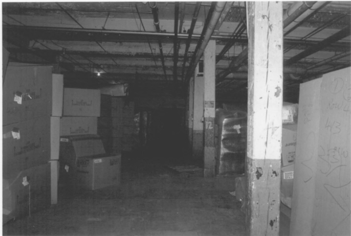
HARDWICK WOOLLEN MILLS BRADLEY COUNTY, TN
