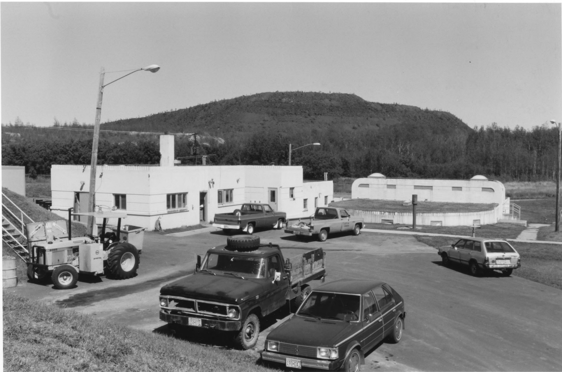
Hibbing Disposal Plant Hibbing, St. Louis County, MN 010829-14
