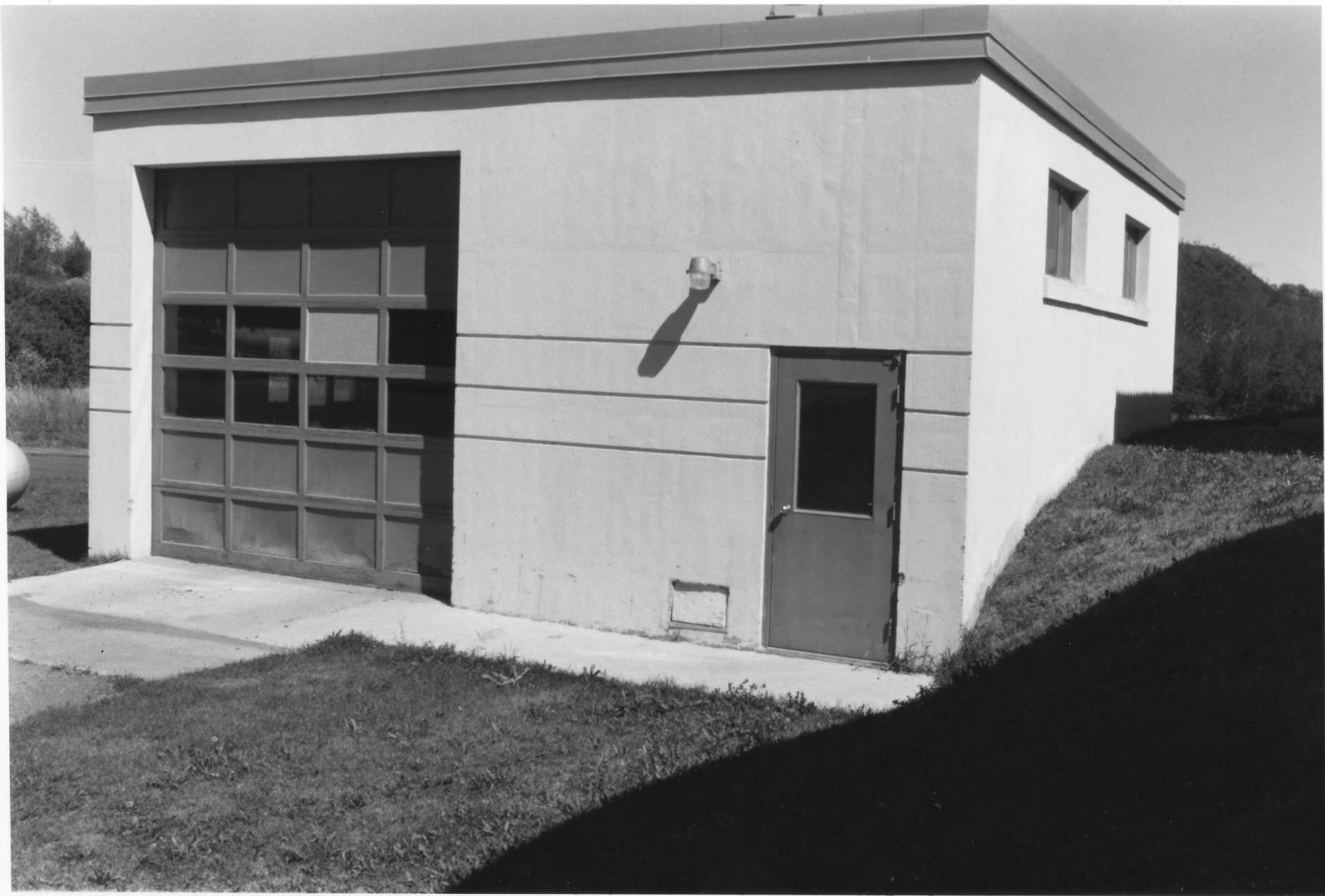
Grit House, Hibbing Disposal Plant (nc) Hibbing, St. Louis County, MN 010829-10A-11
