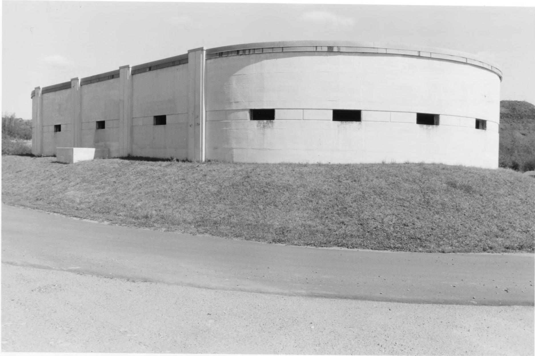
Primary Clarifiers, Hibbing Disposal Plant Hibbing, St. Louis County, MN 010828-16
