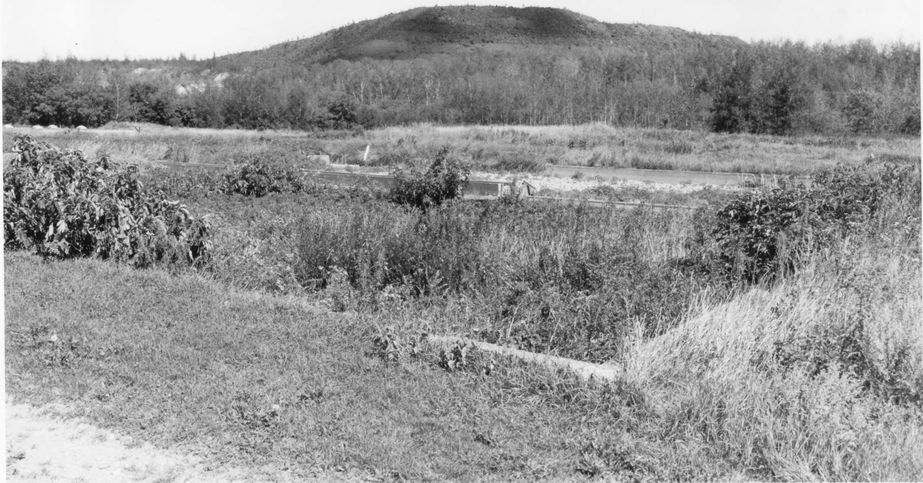
Sludge Drying Bed, Hibbing Disposal Plant Hibbing, St. Louis County, MN 010829-8
