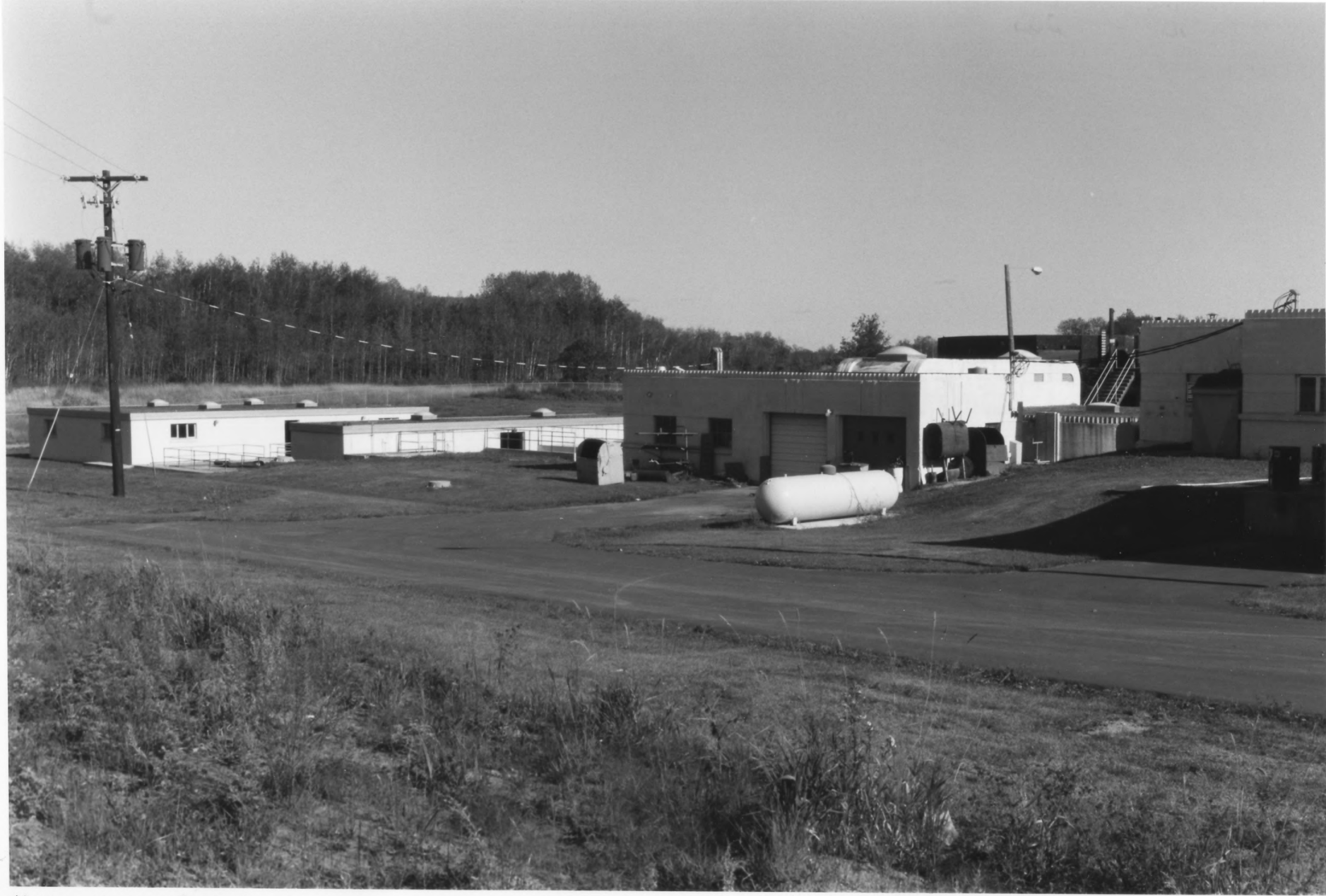
Hibbing Disposal Plant Hibbing, St. Louis County, MN 010829-17A/18
