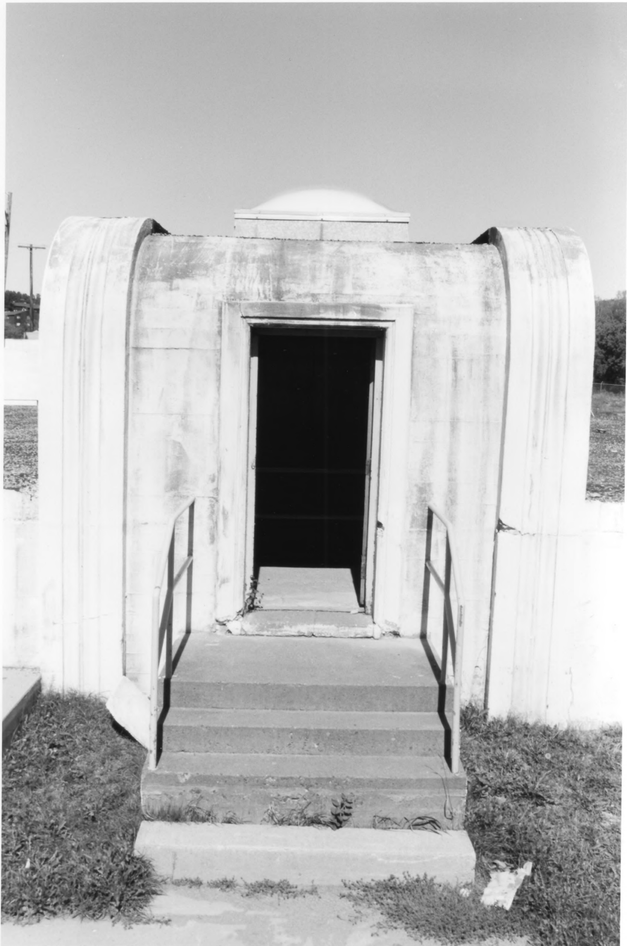
Secondary Clarifiers, Hibbing Disposal Plant Hibbing, St. Louis County, MN 010828-20
