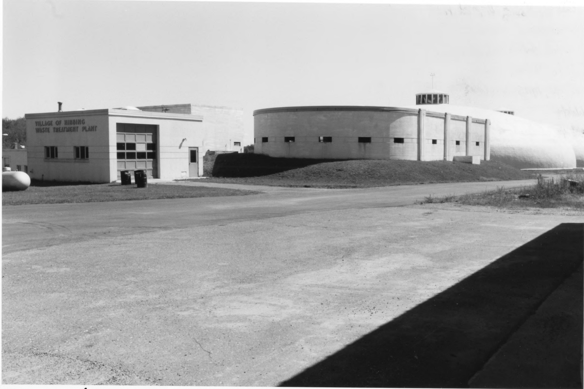
Hibbing Disposal Plant Hibbing, St. Louis County, MN 010829-12
