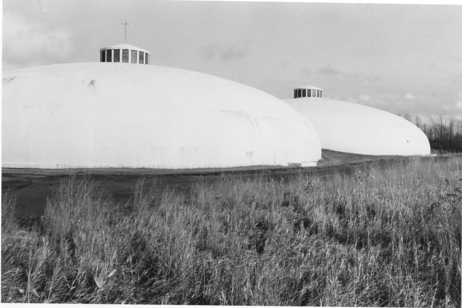
Trickling Filters, Hibbing Disposal Plant Hibbing, St. Louis County, MN
