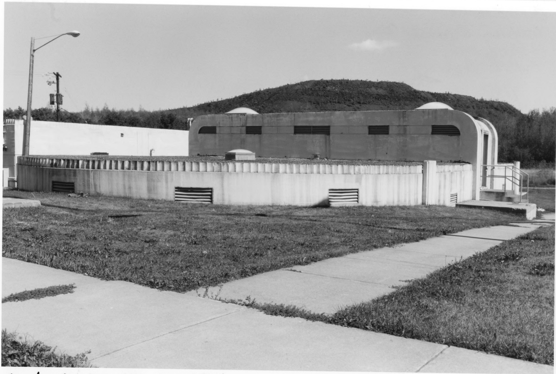
Secondary Clarifiers, Hibbing Disposal Plant Hibbing, St. Louis County, MN
