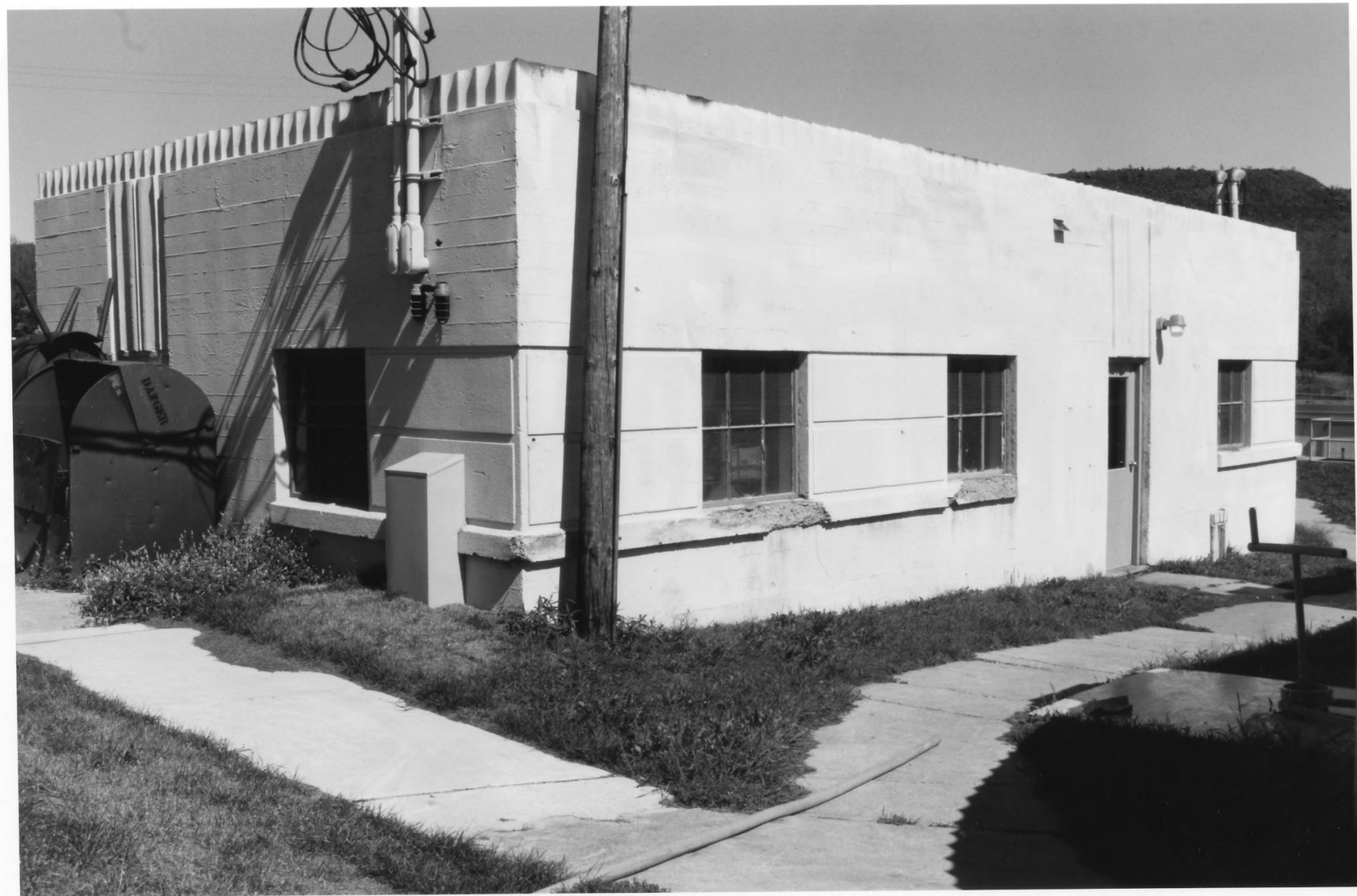
Garage, Hibbing Disposal Plant Hibbing, St. Louis County, MN 010829-3
