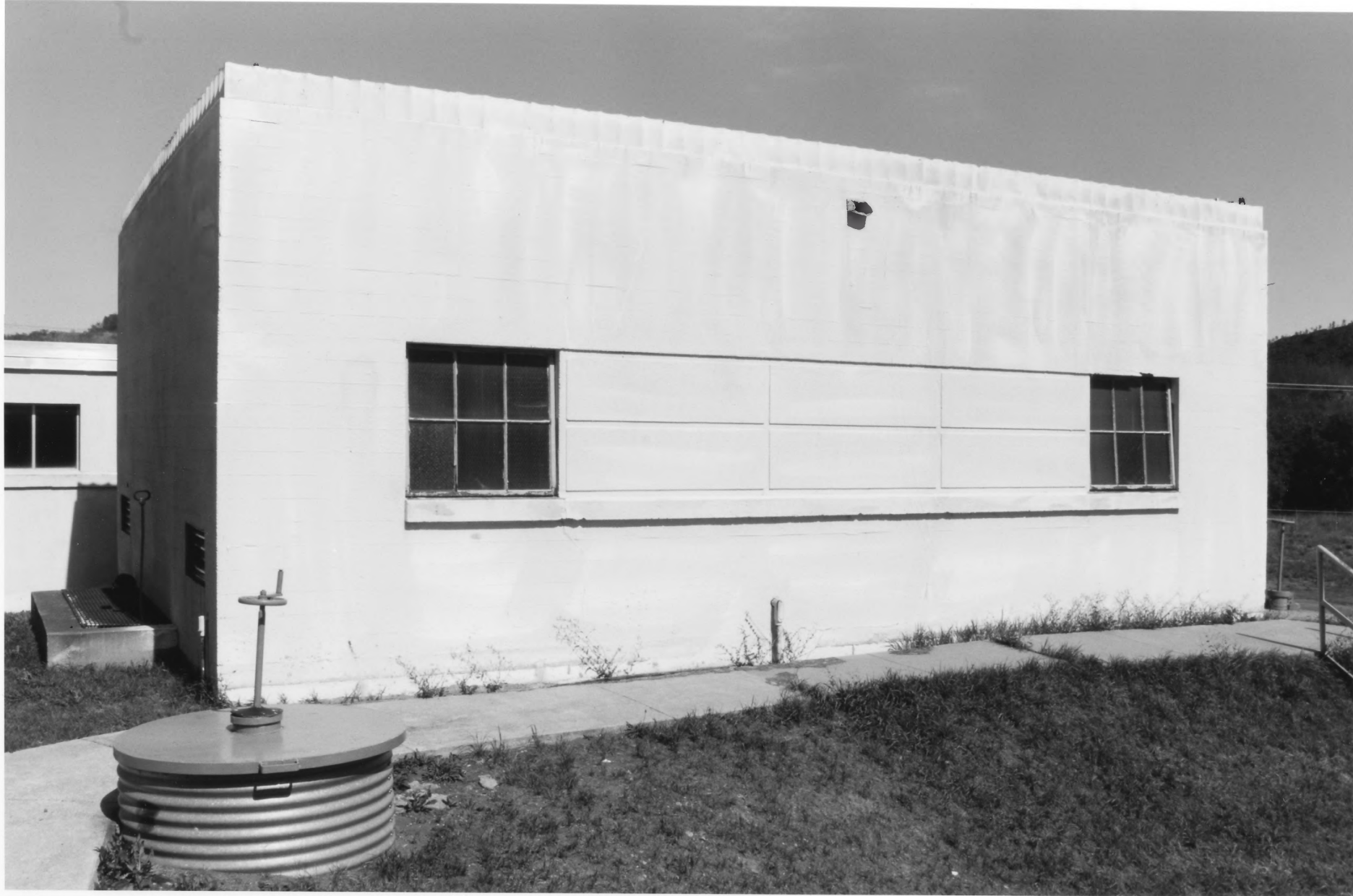
Flocculator, Hibbing Disposal Plant Hibbing, St. Louis County, MN 010828 - 17
