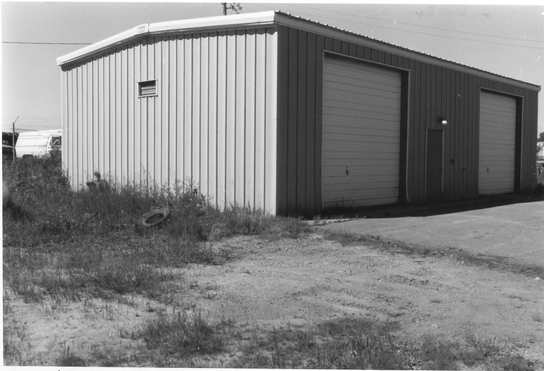
Garage, Hibbing Disposal Plant (nc) Hibbing, St. Louis County, MN 010829 - 9A/10
