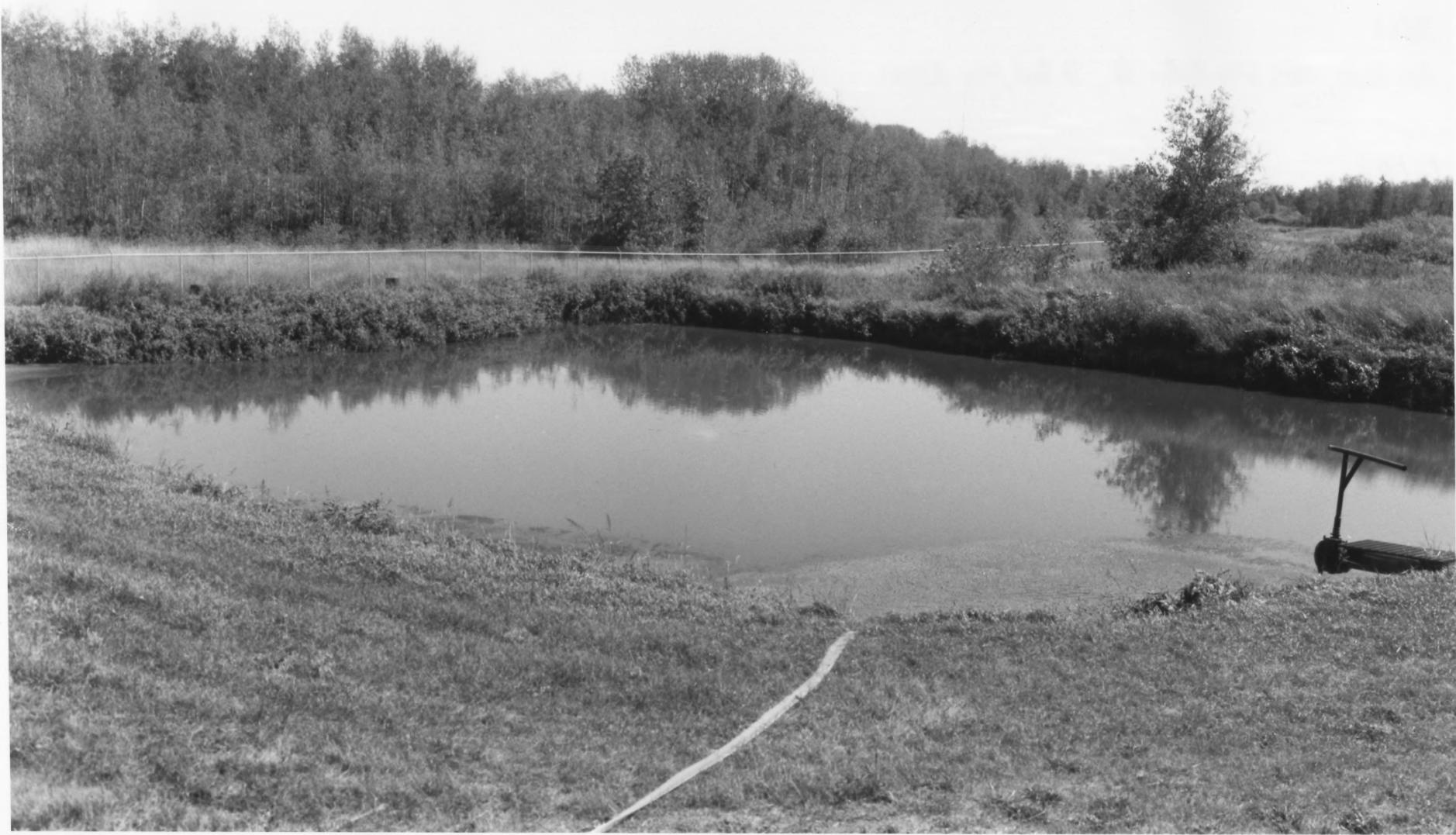
Sludge Lagoon, Hibbing Disposal Plant Hibbing, St. Louis County, MN
