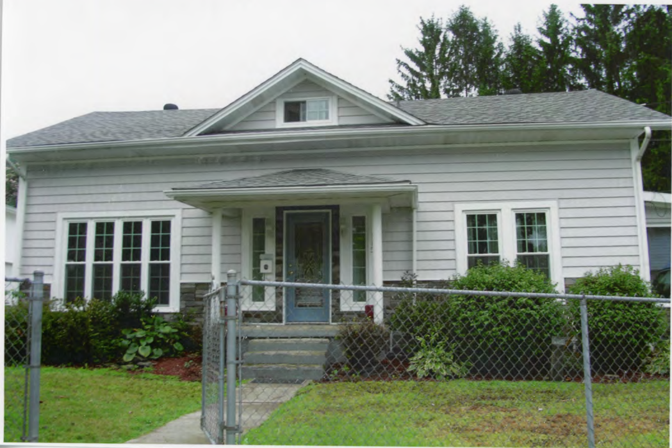
WV - Doddridge County - West Union Res Historic District - 0023
