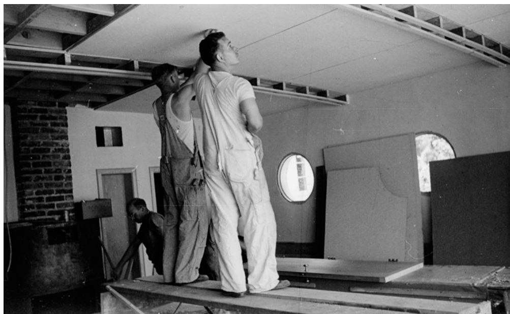
Image 20. Construction – Interior – ca.1938
