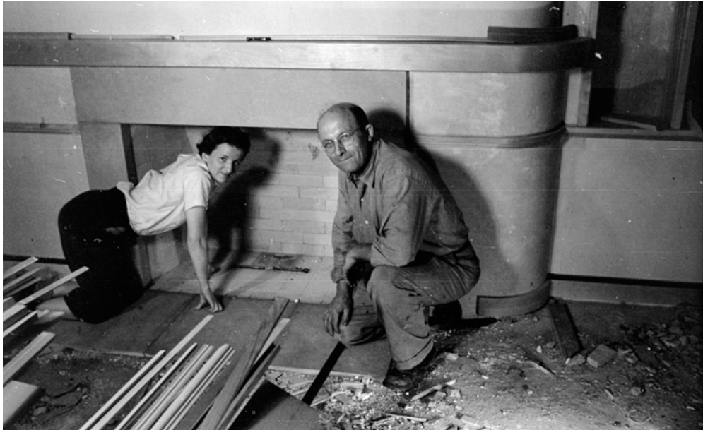
Image 21. Construction – Interior – ca.1938
