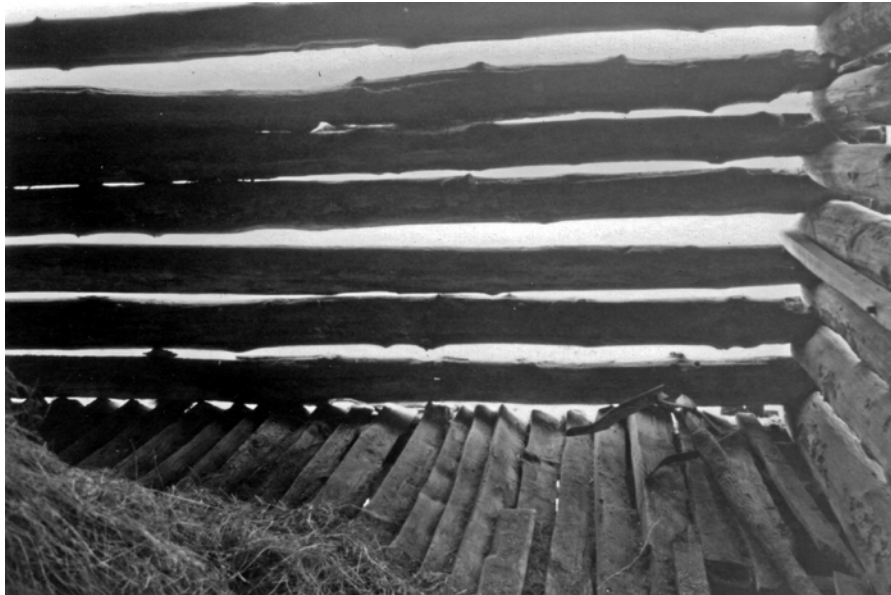
Figure #1 Historic (1981) Log Barn interior: clear view of split rail mow flooring, see photo 21. Camera facing north.
