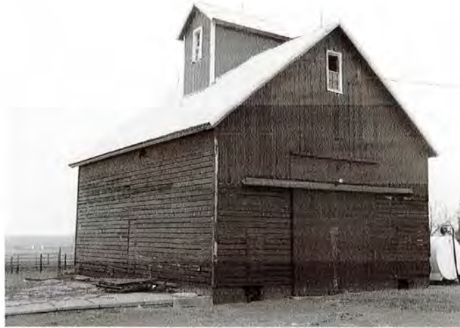
Figure 4 Drive-through slatted corn crib, looking northwest from the central farmstead drive. Bruce Alleman photo, 2014.
