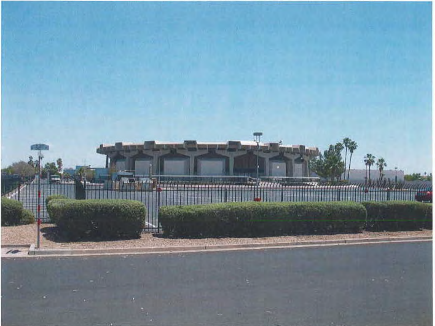
Photograph 1. The theater from the corner of 32 nd Street and Fillmore Street, facing southwest.
