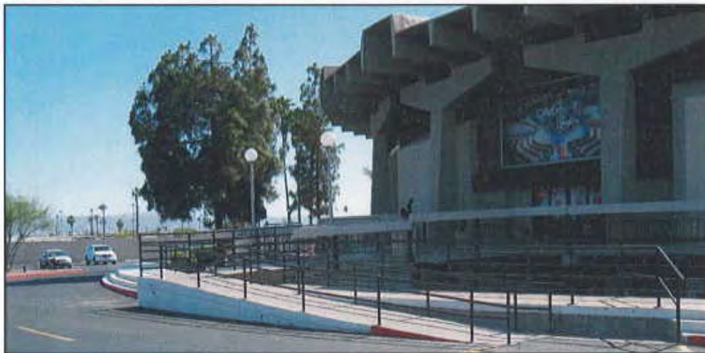
Figure 5. The accessibility ramp and east moat bridge, facing southwest.
