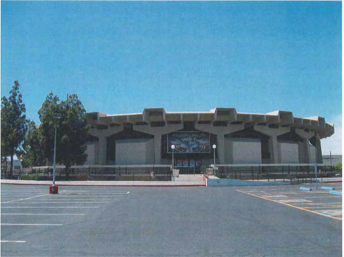
Photograph 2. East entrance, facing west.
