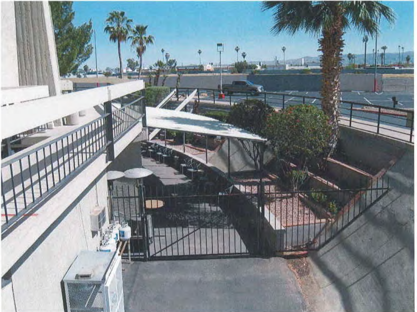
Photograph 7. Covered patio area in moat, facing southeast.
