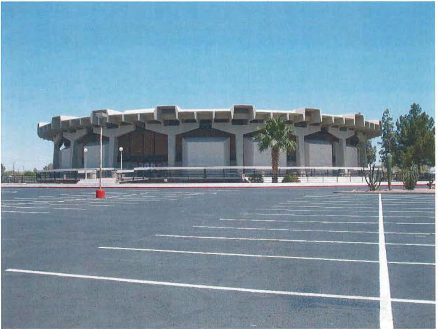
Photograph 4. West entrance facing northeast.
