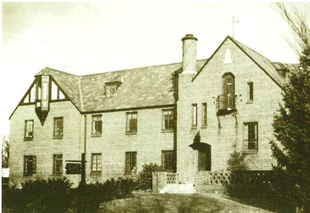
1937 BUILDING PHOTO Figure No. 13
