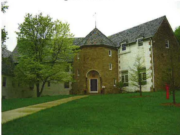
View of original house (constructed in 1931) from Gray Avenue - East View
