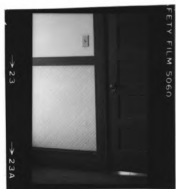
Fig. 4g detail of front bedroom facing south
