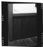
Fig. 4f detail of old kitchen facing east
