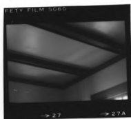
Fig. 4d living room ceiling facing NE
