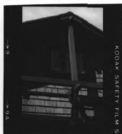
Fig. 4b detail of roof support facing west
