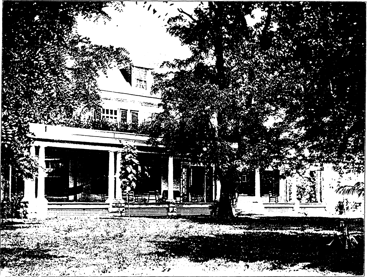
Front Elevation of Residence.
