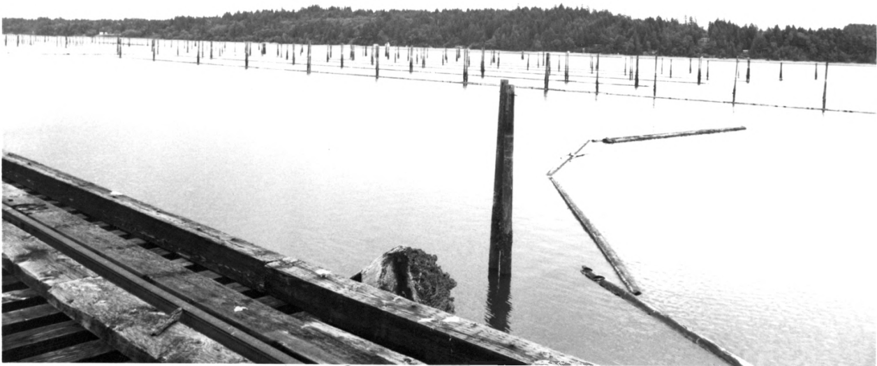
CATWALKS AND DOLPHINS/WSBLDRHDL OLYMPIA, WASHINGTON
