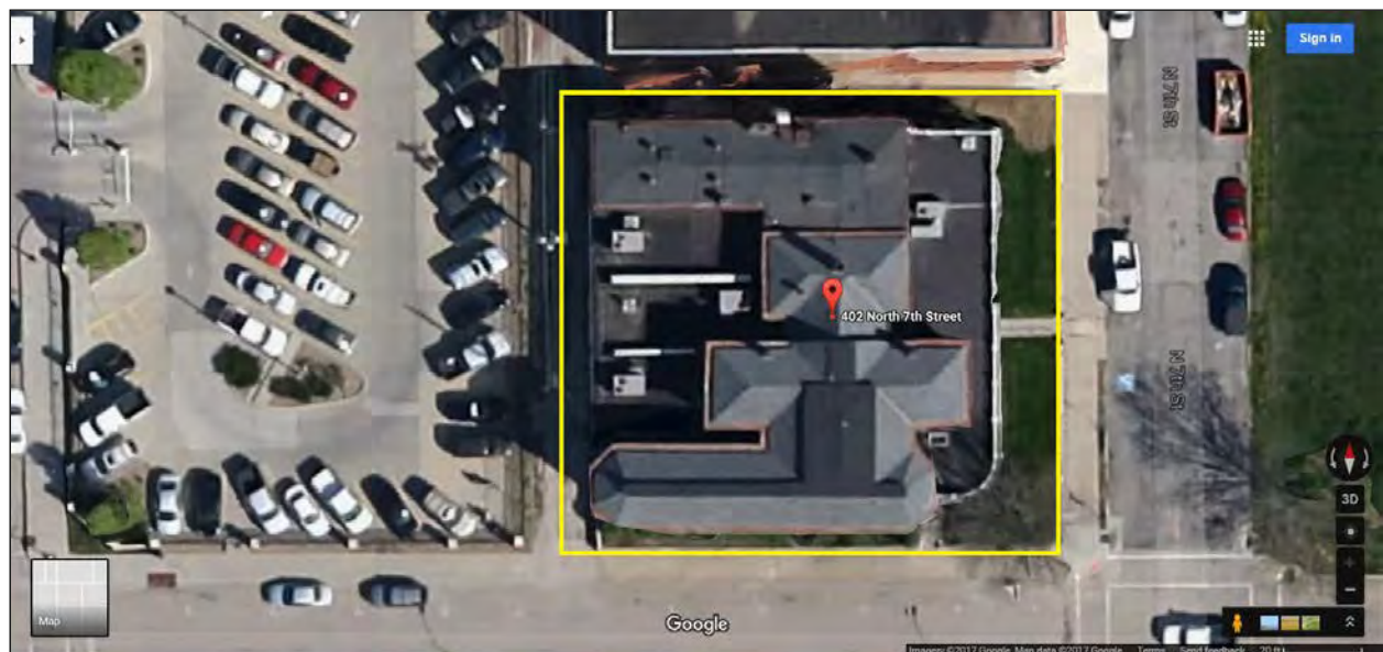
Figure #04 Google Map – Earth view of The Benton Club building (police parking lot to the west). The Benton Club location is marked and bounded by yellow. https://www.google.com/maps/place/402+N+7th+St,+St+Joseph 402 N 7 th Street, St. Joseph, Missouri 64501 39°46'09.3"N 94°51'08.1"W
