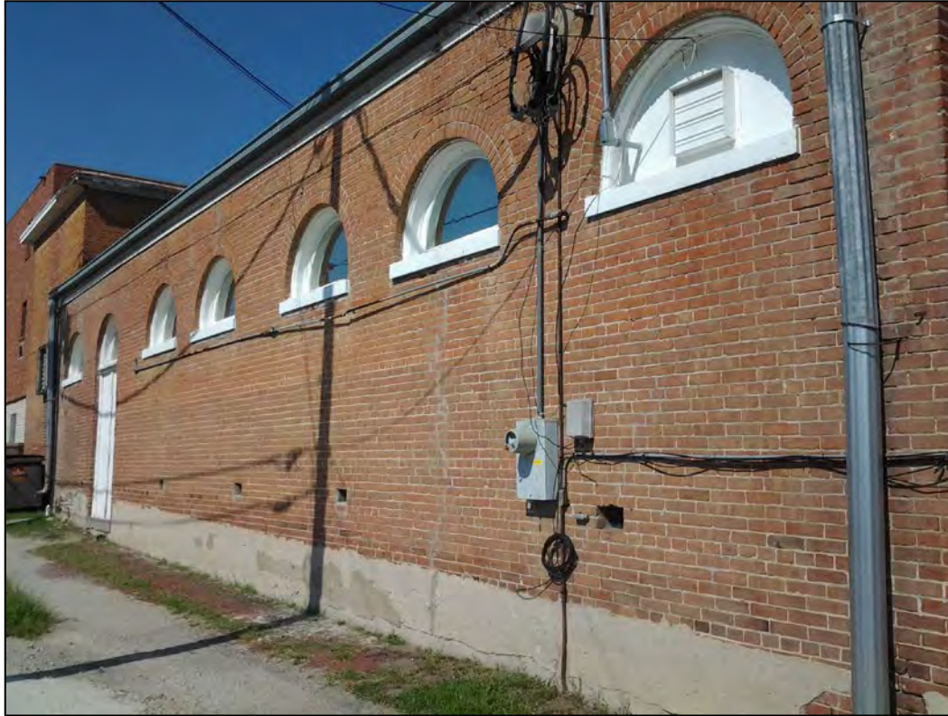
Figure F14. View of west side of building showing arched windows and double door. Camera is pointed northeast.
