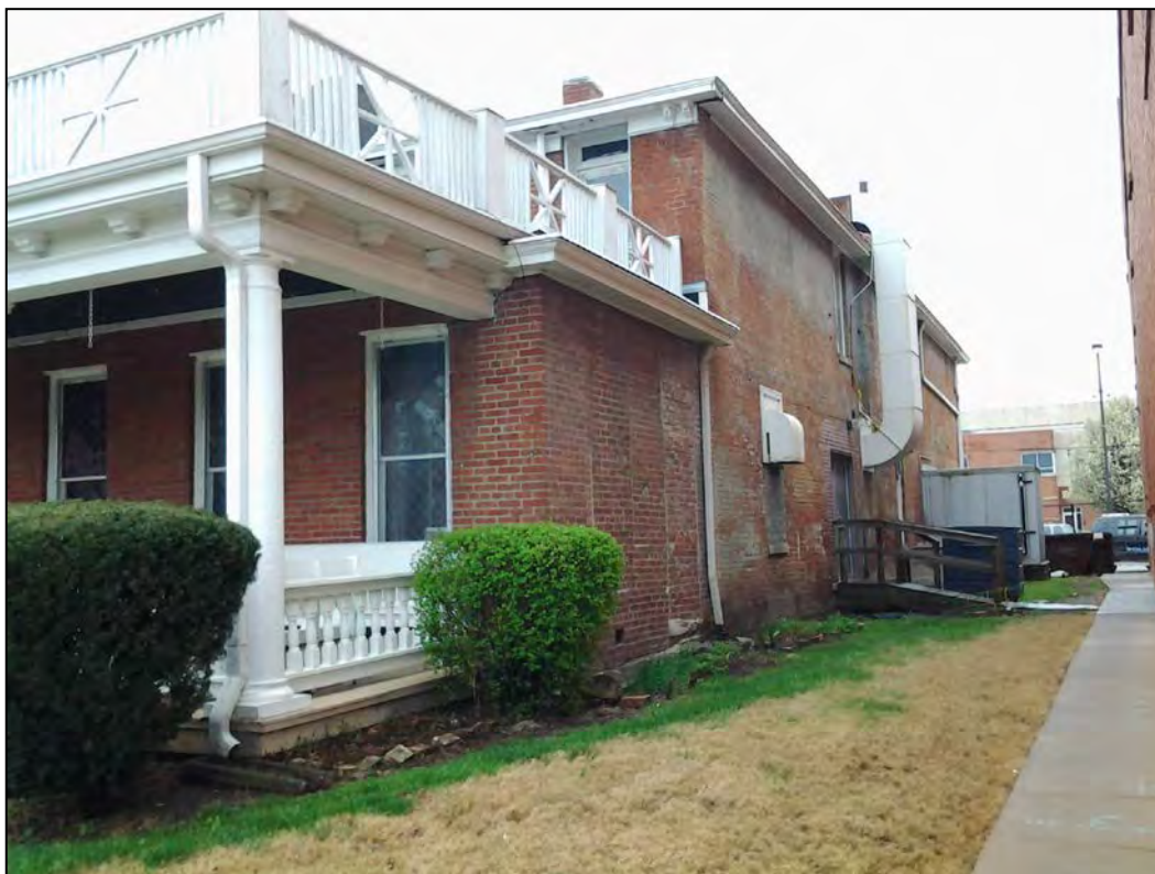
Figure F15. View of kitchen door on north side of building with ramp. Camera is pointed southwest.
