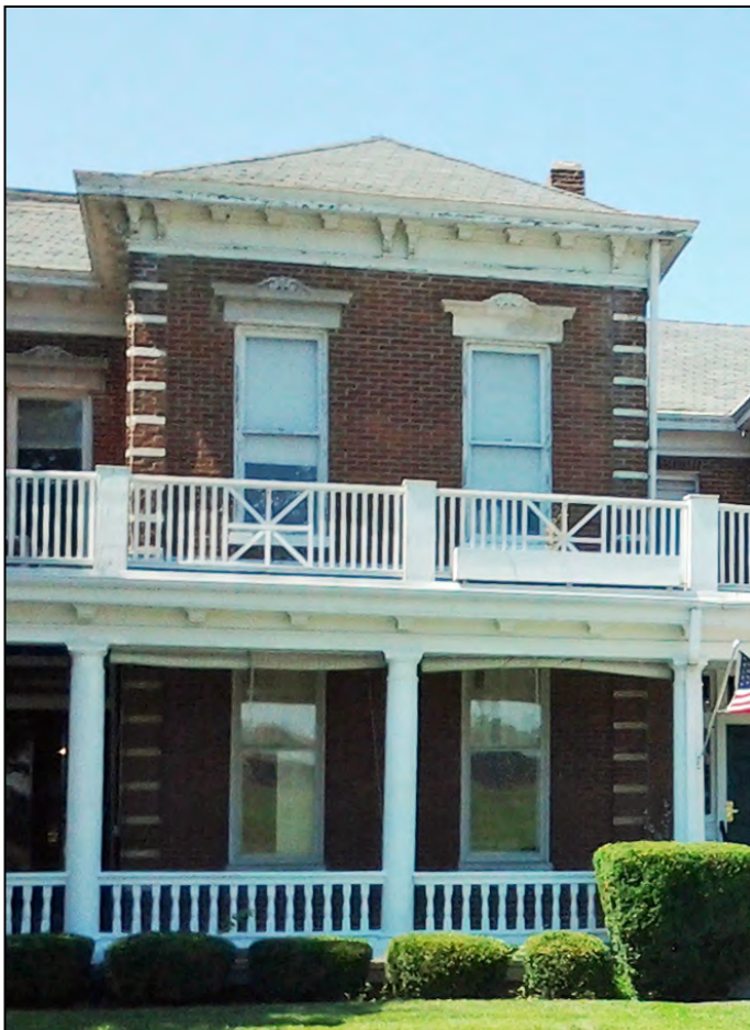
Figure F13. View of structure showing decorative quoins and wooden brackets on eaves. Camera is pointed west.
