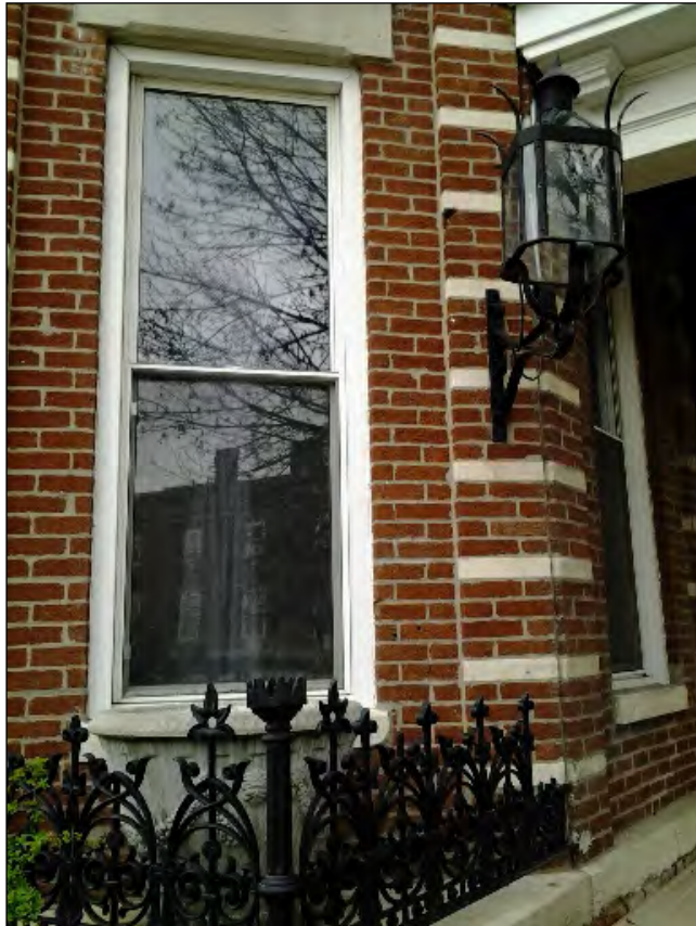
Figure F10. View of south entrance to the porch, with wrought iron decorations. Camera is pointed north-northwest.
