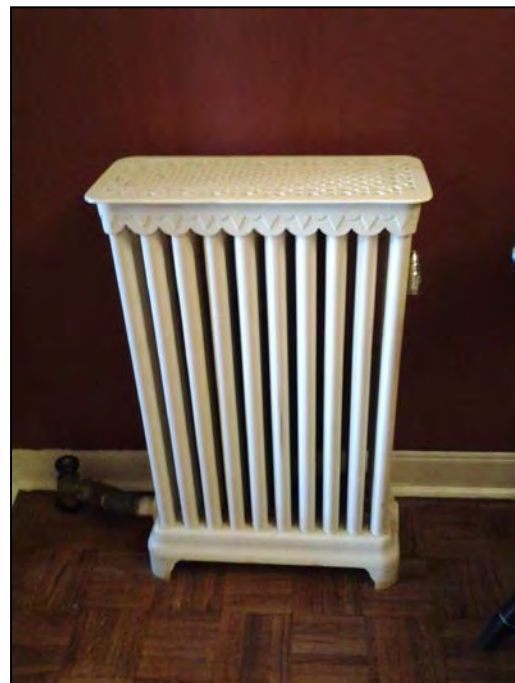
Figure F27. An original radiator still located in the entry hall.
