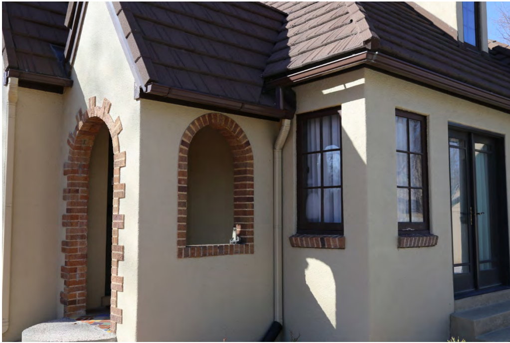
Photograph 5 South and east elevations of house, porch details. Camera facing northwest.
