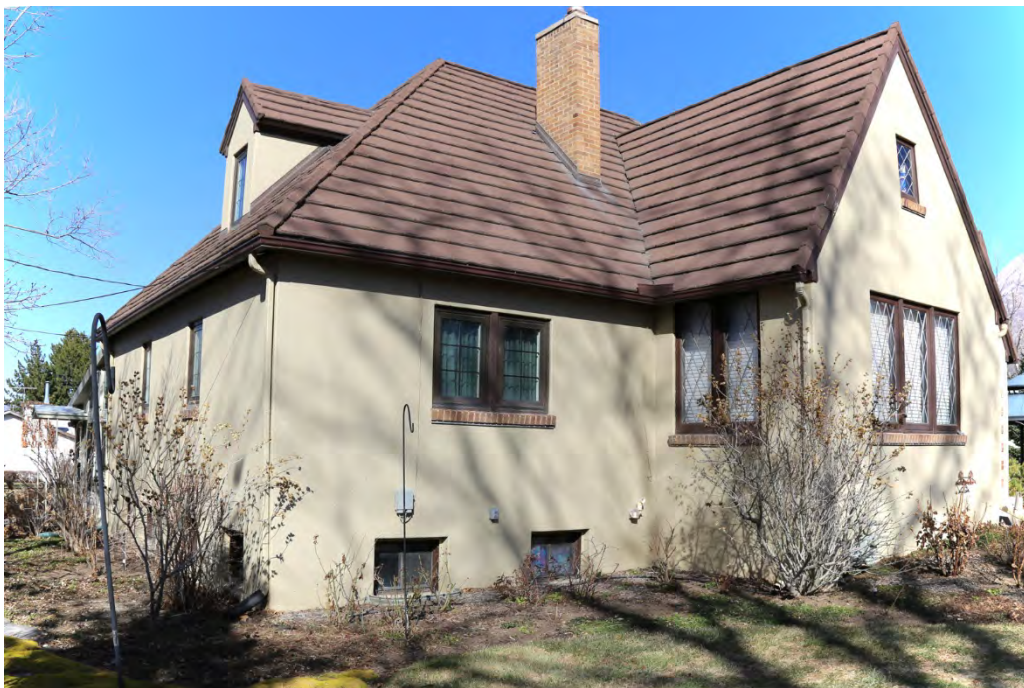
Photograph 4 South and west elevations of house. Camera facing northeast.
