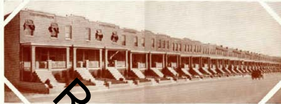
View of 24th Street Looking South to Government Property
