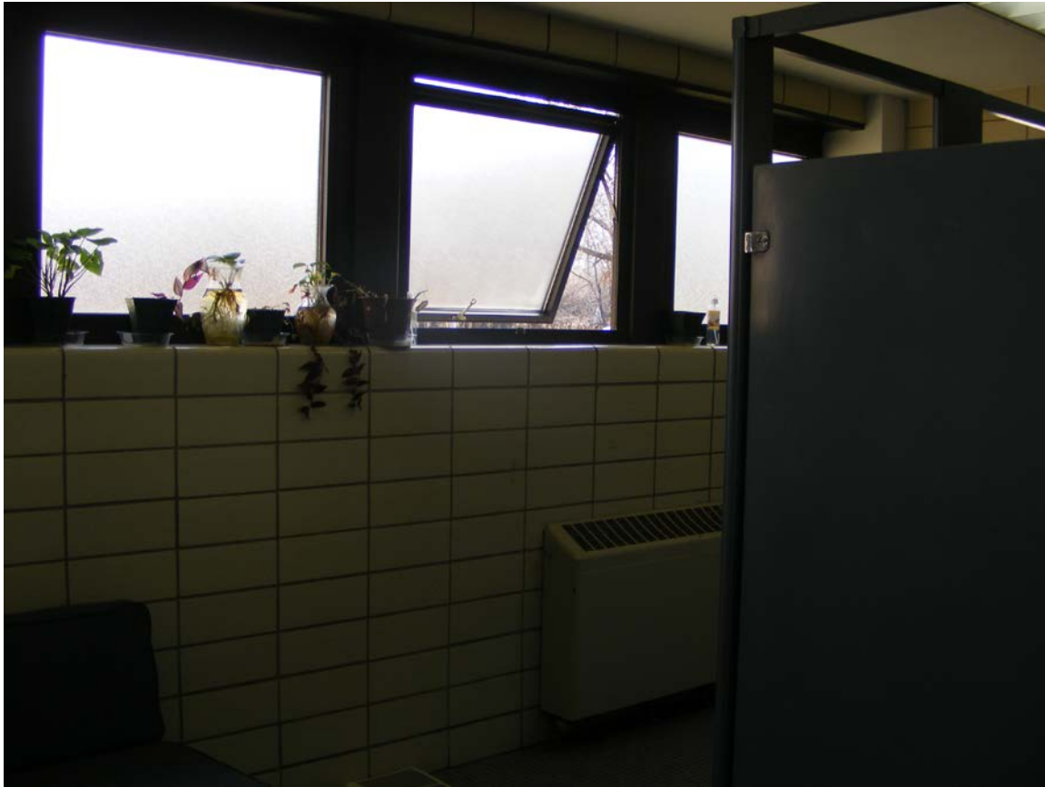
Figure 10. Wrapped windows retain original aluminum framing, as illustrated by the open window in this photograph (Photo: Ruth Keenoy).
