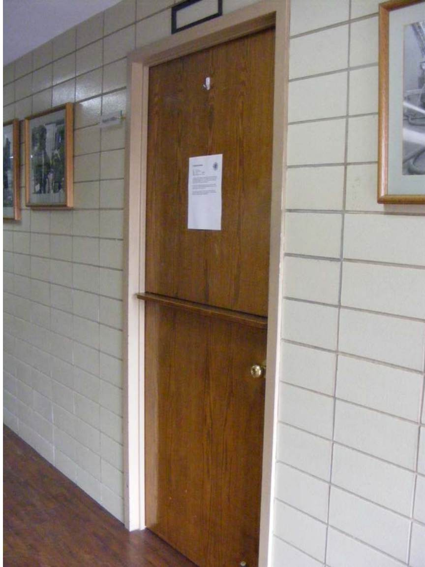
Figure 9. Original exam room door, view is northeast (Photo: Ruth Keenoy).
