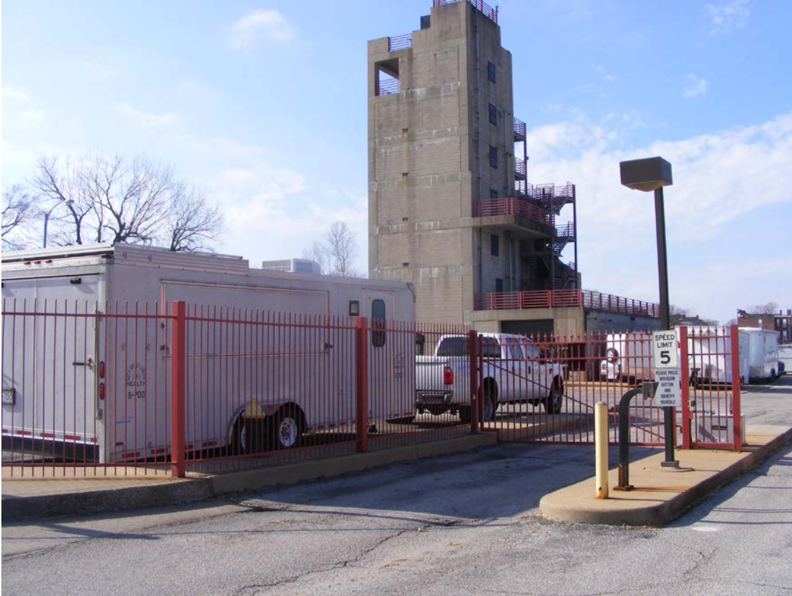
Figure 6. The parking lot, practice tower and associated entry gate/drive south of the former health clinic are outside of the property's National Register boundaries (Photo: Ruth Keenoy).
