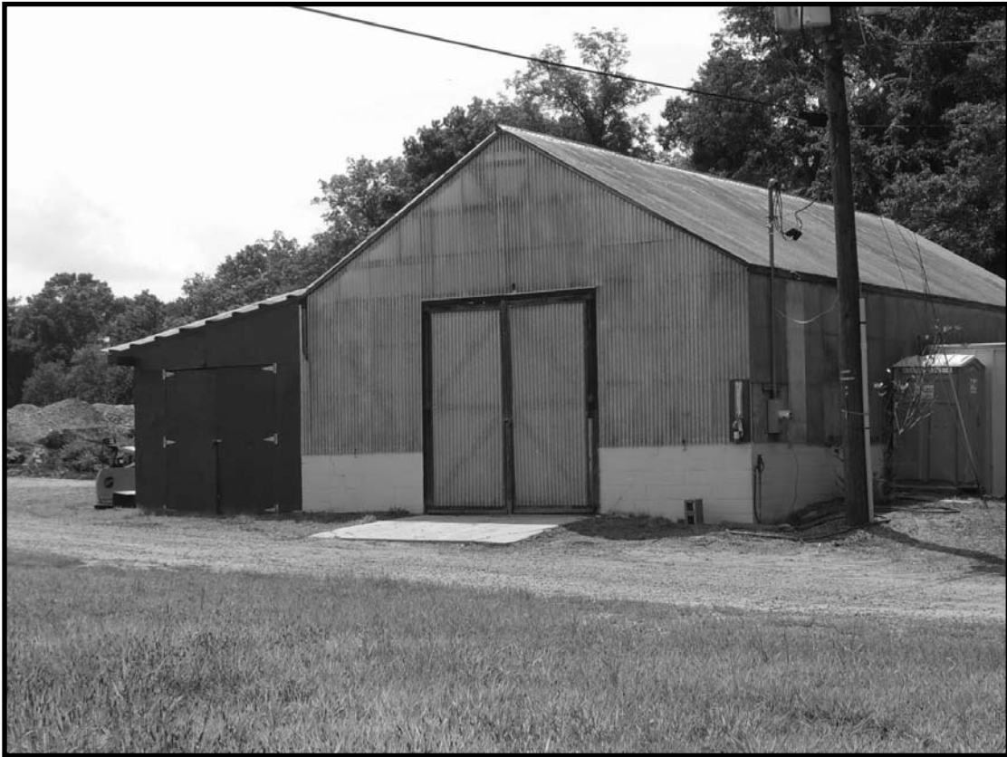
Princeton Nurseries Historic District, Plainsboro and South Brunswick Townships, Middlesex County, New Jersey
