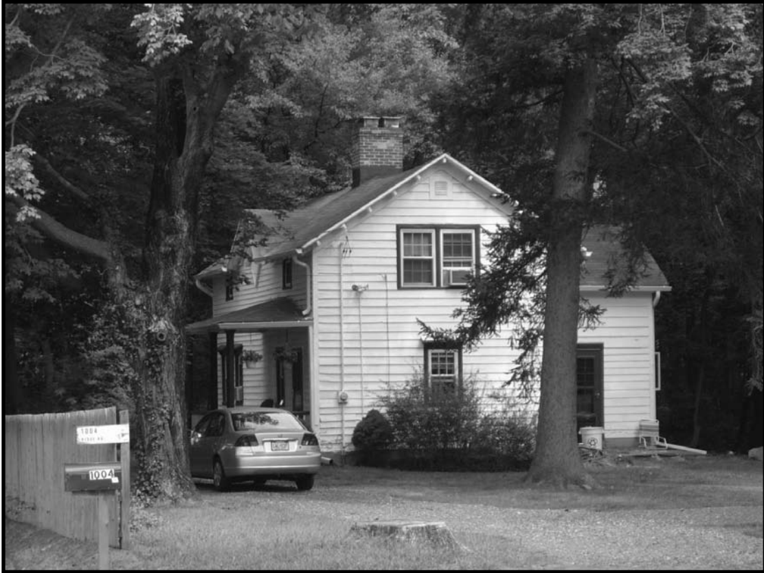
Princeton Nurseries Historic District, Plainsboro and South Brunswick Townships, Middlesex County, New Jersey
