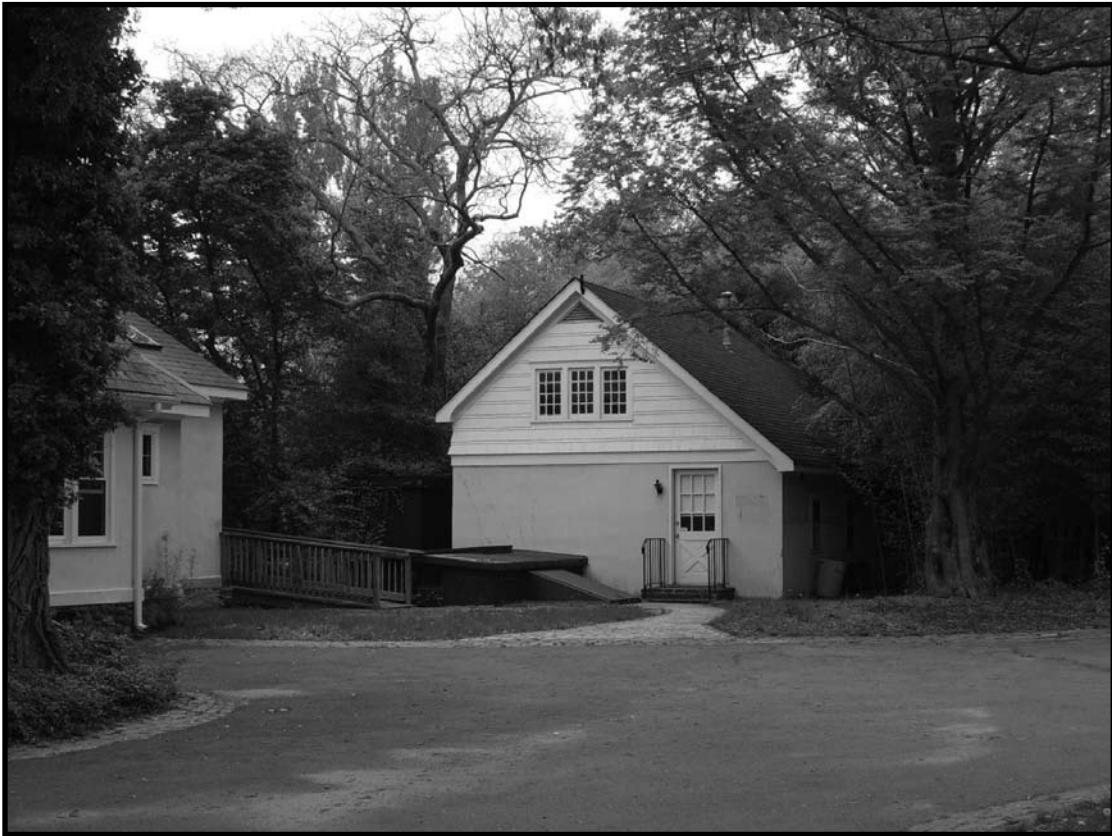
Princeton Nurseries Historic District, Plainsboro and South Brunswick Townships, Middlesex County, New Jersey
