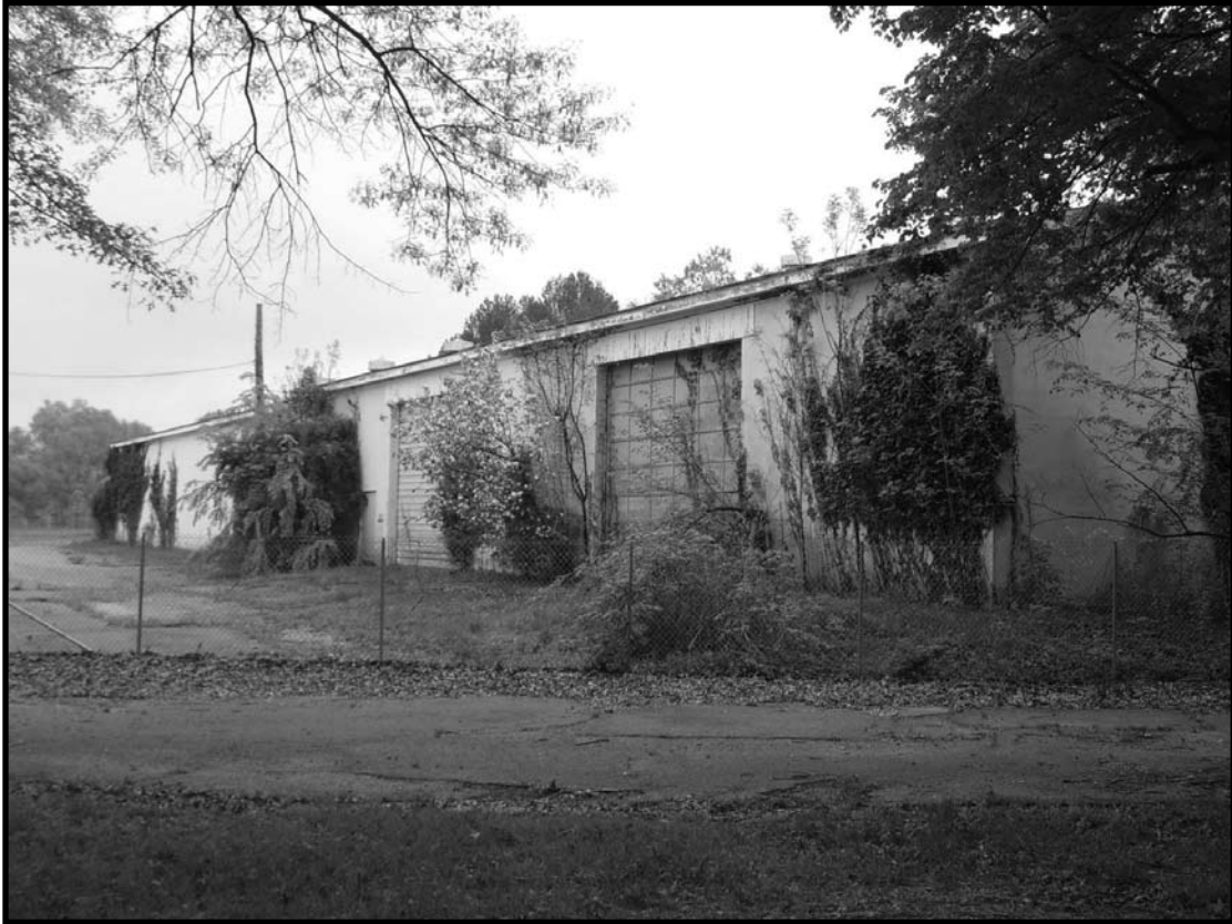
Princeton Nurseries Historic District, Plainsboro and South Brunswick Townships, Middlesex County, New Jersey
