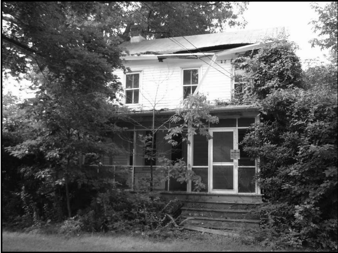
Princeton Nurseries Historic District, Plainsboro and South Brunswick Townships, Middlesex County, New Jersey
