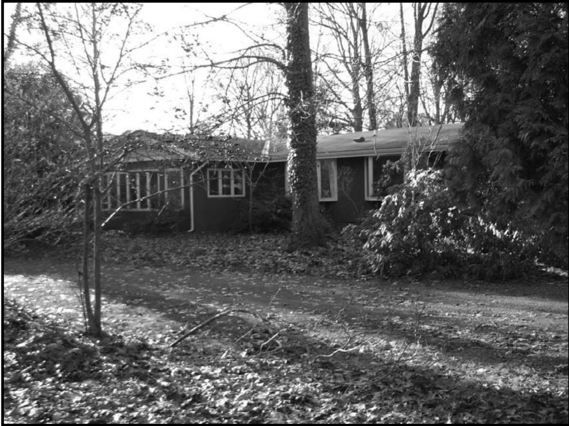
Princeton Nurseries Historic District, Plainsboro and South Brunswick Townships, Middlesex County, New Jersey
