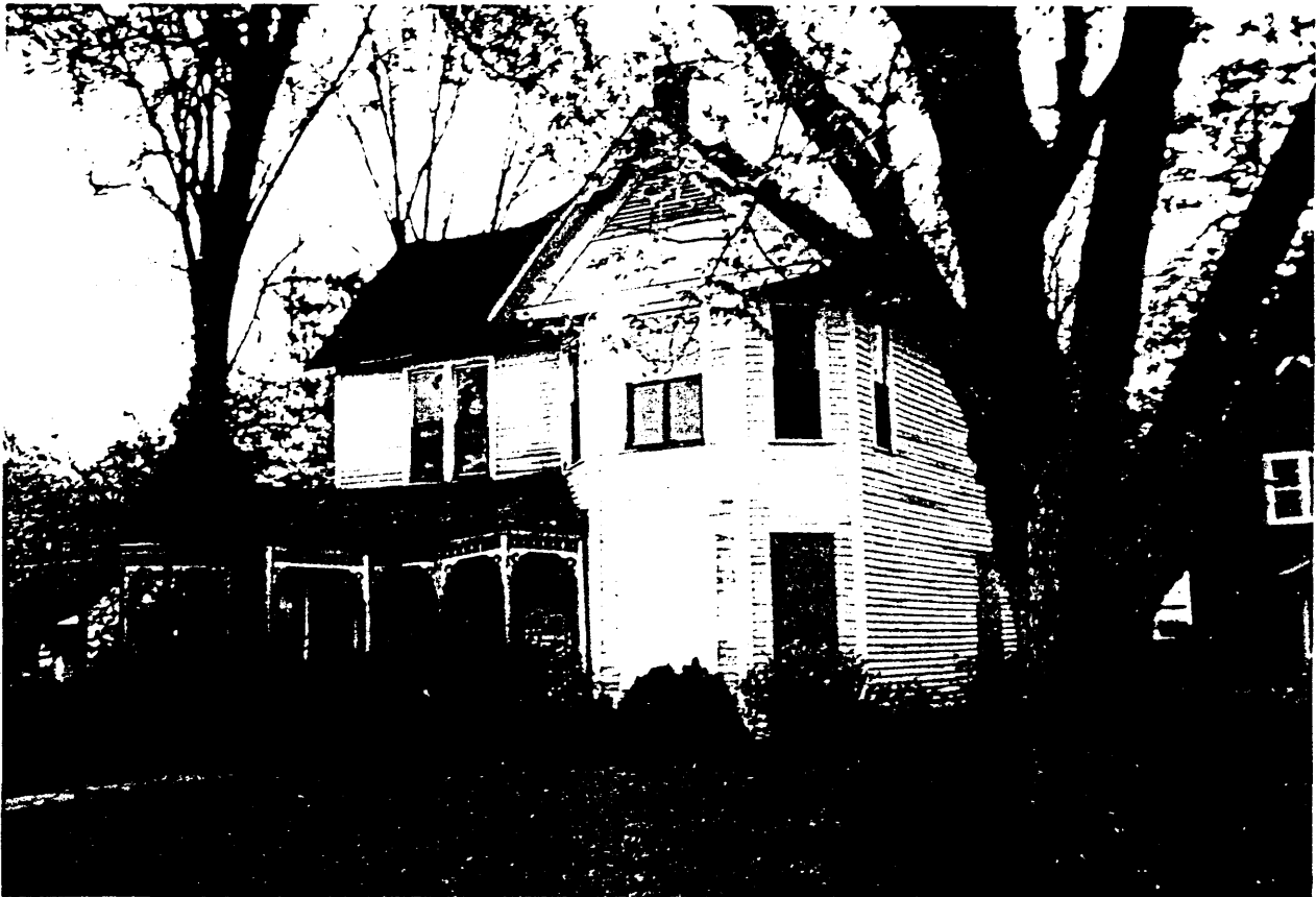
Photograph Before Renovations #2 of 4: Caldwell-Hopson House
