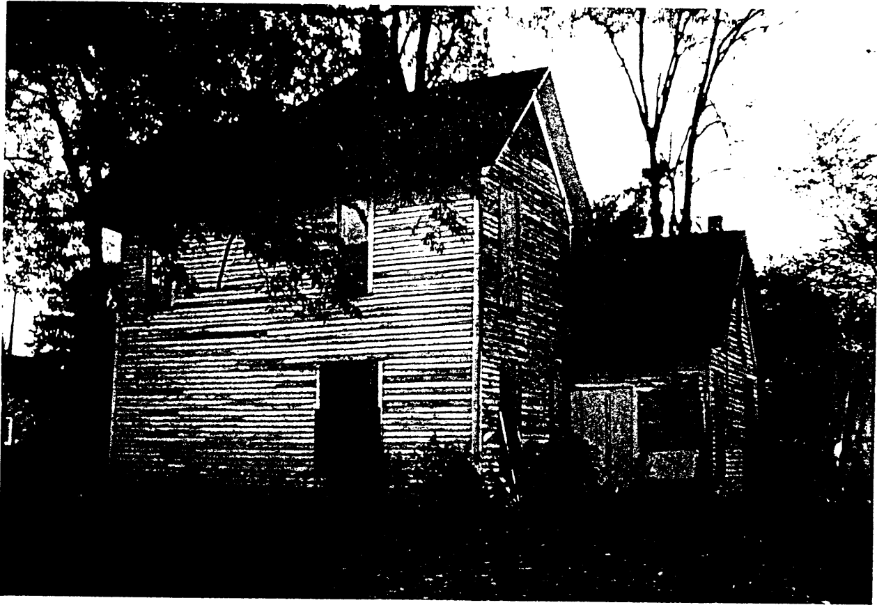
Photograph Before Renovations #3 of 4: Caldwell-Hopson House
