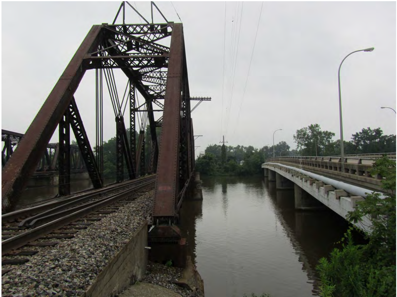
Photo 5. View to the south of railroad bridges and Dixie Highway crossing the River Raisin. This transportation corridor follows the route north from Frenchtown that was laid out by General William Hull in 1812.
