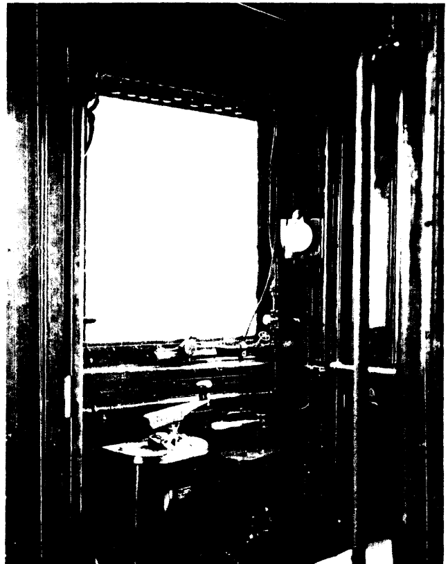
The engineer's cab in the vestibule of the M. U. has an air brake lever, speed controller, whistle rope, and on the floor a dead man's pedal. Above the window are push buttons for raising and lowering the pantographs, turning on the headlights, and operating several electrical controls.
