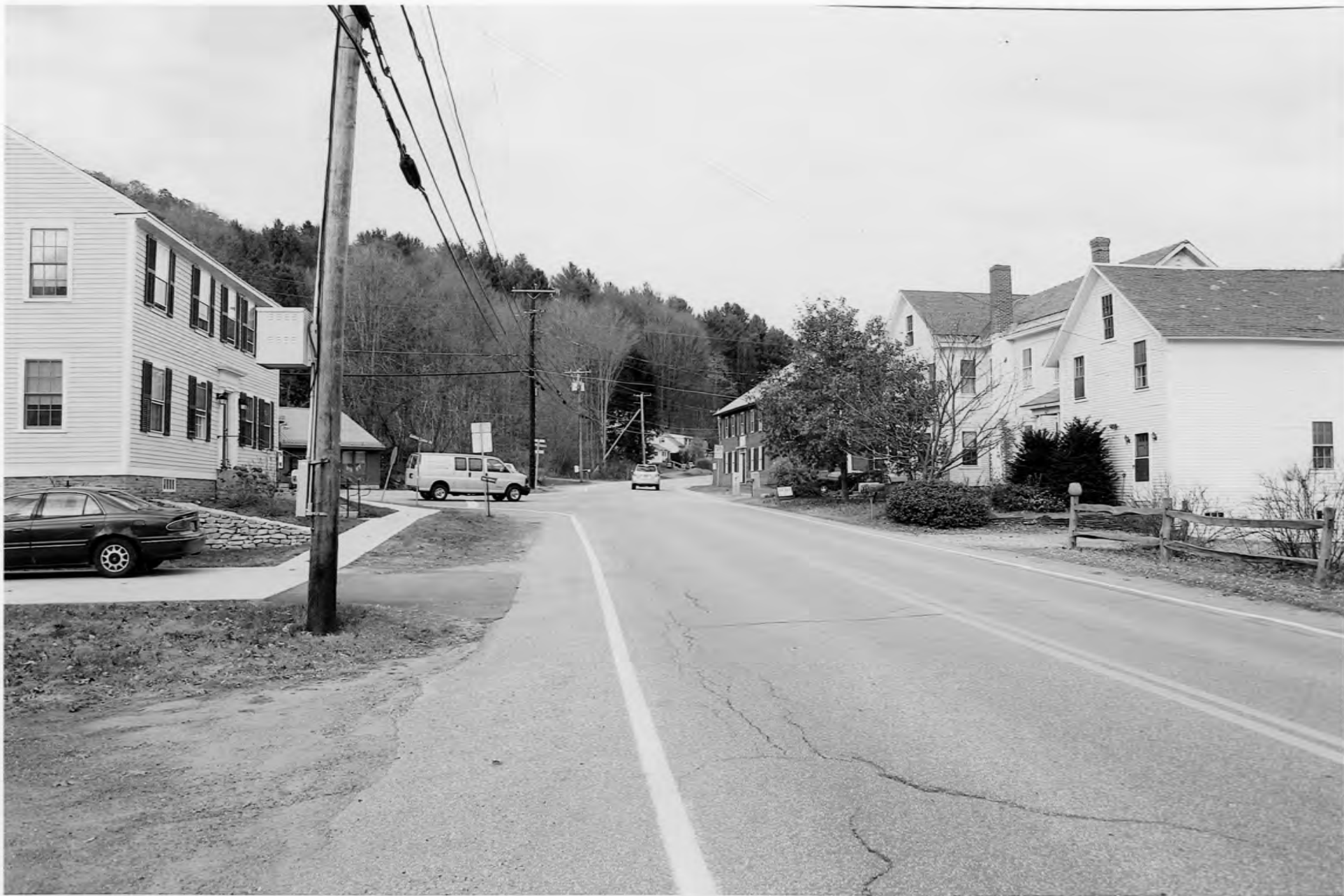
Broad Brook House; Guilford, Windham Co., VT (11/1/2010 by L. Papazian, Digital images are on file at the Vermont Division for Historic Preservation) Photo. #3 of 10: View of Algiers Village with Broad Brook House (center right), & Tontine Bldg. (left), looking north on U.S. Route 5/Coolidge Hwy
