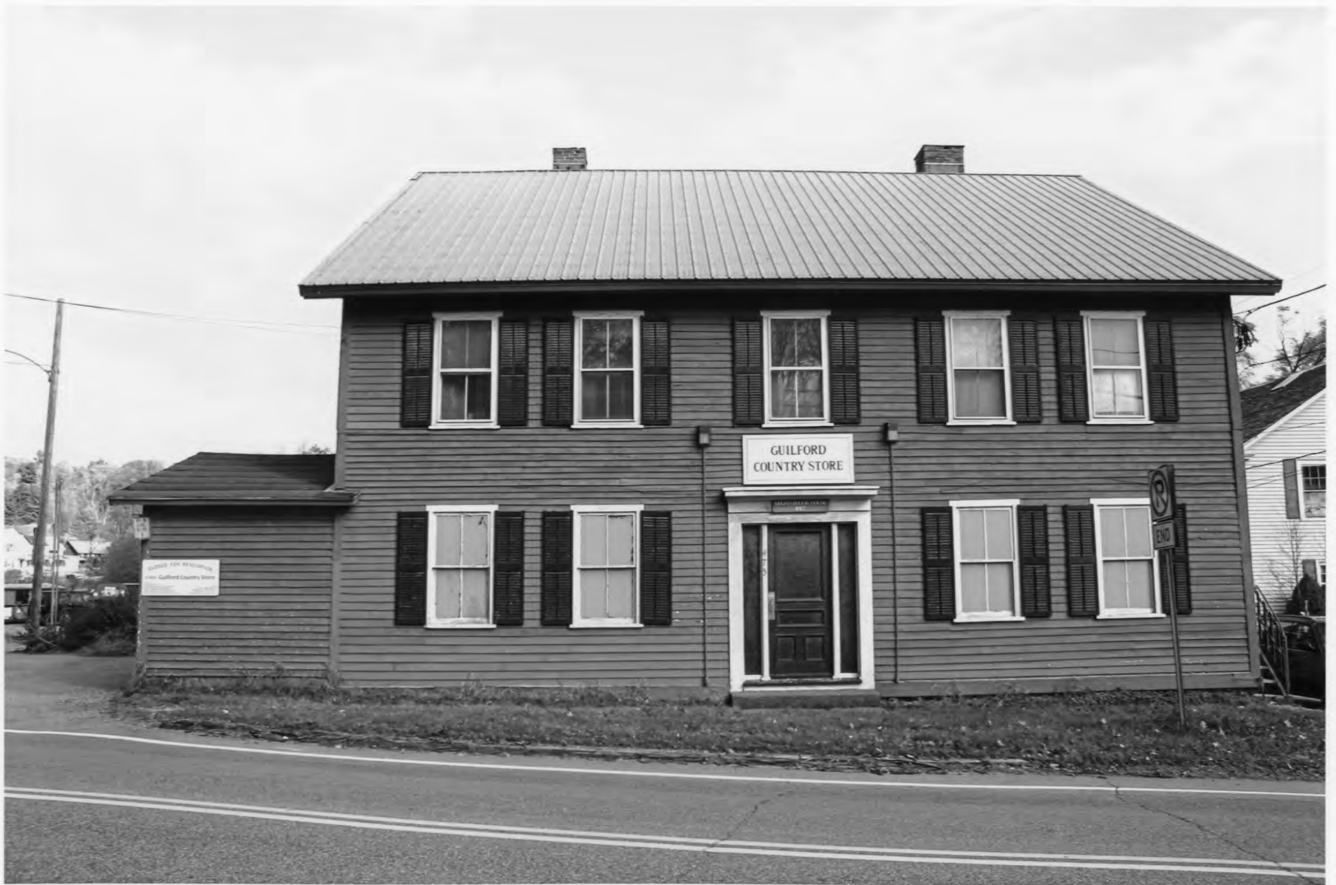
Broad Brook House; Guilford, Windham Co., VT (11/1/2010 by L. Papazian, Digital images are on file at the Vermont Division for Historic Preservation) Photo. # 5 of 10: View looking east of front (west) facade
