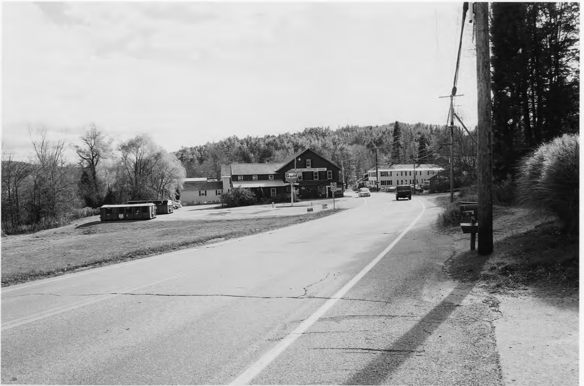
Broad Brook House; Guilford, Windham Co., VT (11/1/2010 by L. Papazian, Digital images are on file at the Vermont Division for Historic Preservation) Photo. #2 of 10: View of Broad Brook House (left), Tontine Bldg. (right) & Algiers Village, looking south on U.S. Route 5/Coolidge Hwy
