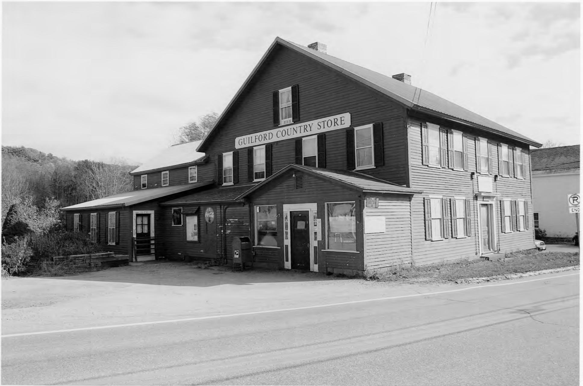
Broad Brook House; Guilford, Windham Co., VT (11/1/2010 by L. Papazian, Digital images are on file at the Vermont Division for Historic Preservation) Photo. #4 of 10: View looking southeast of north and west (front) facades
