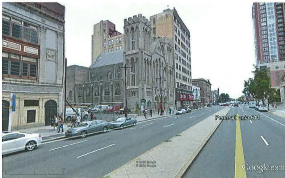
Figure 29: Chambers-Wylie Presbyterian Church, 321 S. Broad Street, 1899-1901, Rankin & Kellogg, architects. Source: Google Earth
