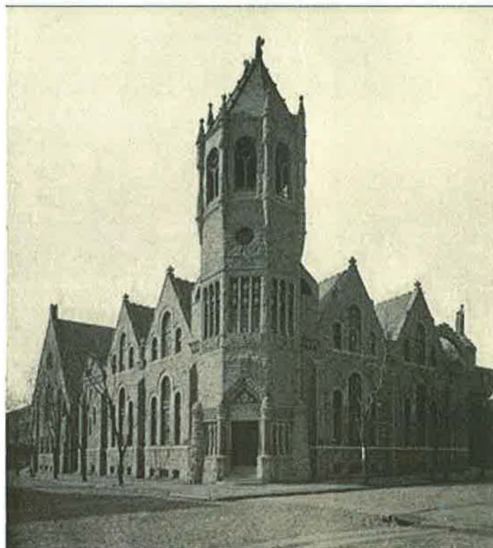
Figure 21: West Hope Presbyterian Church., 4052 Aspen St., 1890, T. Frank Miller, architect. Source: White and Scott, courtesy Philadelphiabuildings.org.
