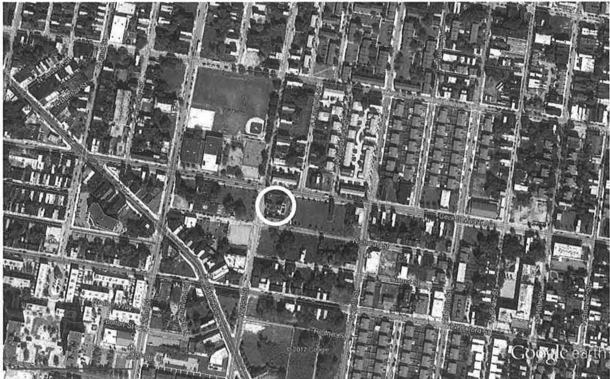
Figure 1: Google Earth view, showing McDowell Memorial Presbyterian Church (in circle) and setting
