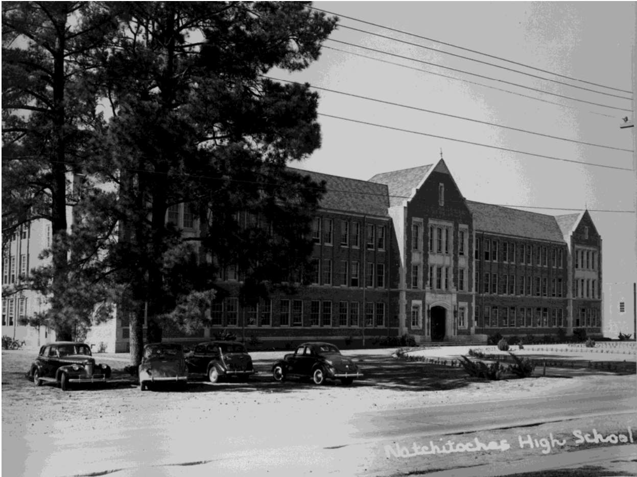
Figure 5. Historic Image of Natchitoches High School. Courtesy of: F1804, Cammie G. Henry Research Center, Watson Memorial Library, Northwestern State University of Louisiana.
