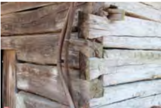
Photo 0013 corner construction of smokehouse
