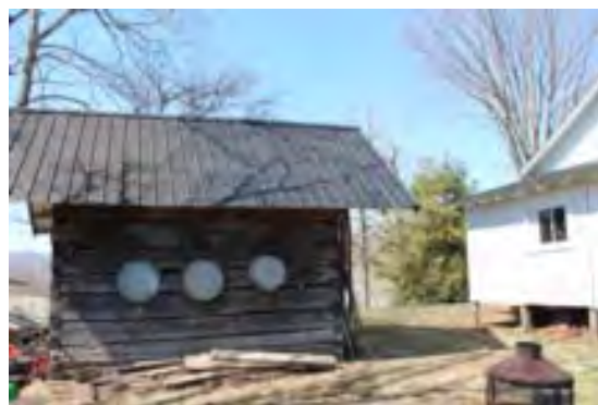
Photo 12: East side, Smokehouse
