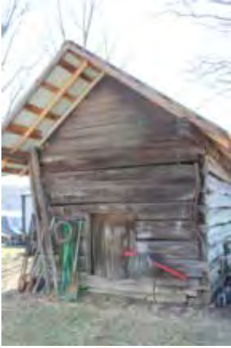
Photo 0011 view of NE front of smokehouse
