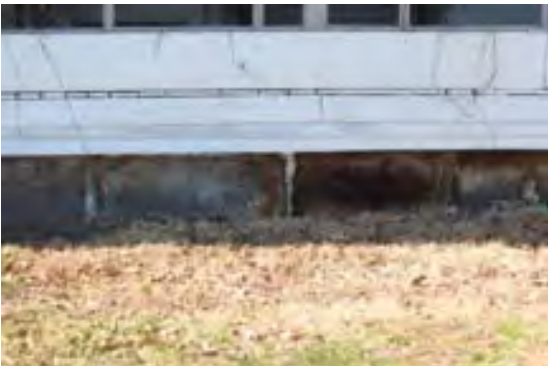
Photo 0010 view of house foundation
