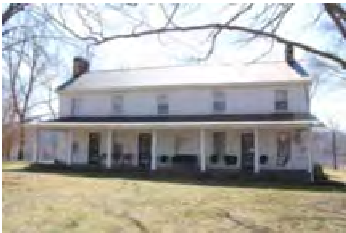
Photo 6, front of original house
