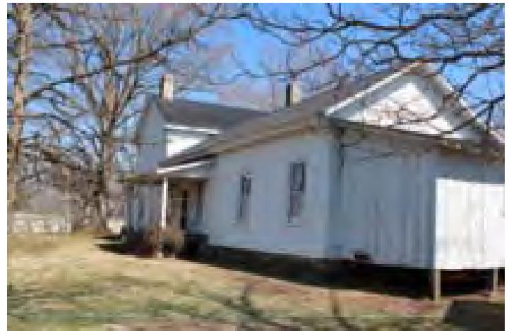
Photo 7, view of Southwest side of house
