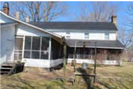
Photo 0008 rear view of the house
