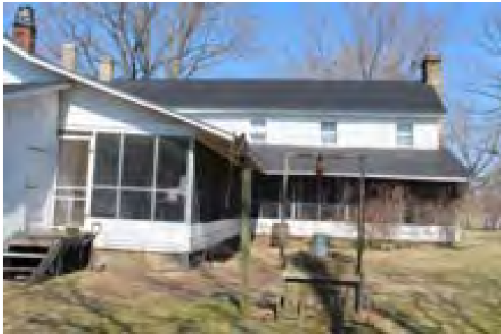
Photo 8: Rear view of the House
