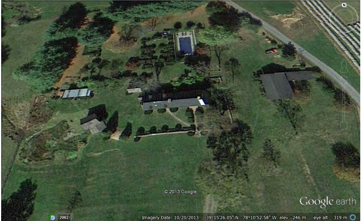
Figure 1: Aerial View of the Springdale Property using Google Earth (close-up of House and outbuildings on 4.46 acres)
