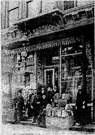
J. Schmuck Block's original storefront, 1887
