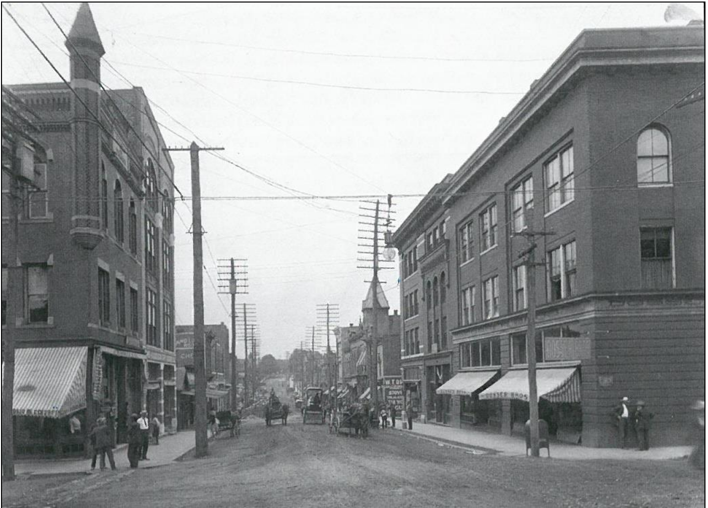
Figure 5. 1910 view of Main Street taken from just east of Cumberland Street intersection. Myers Building (#20) can be seen at left and was built circa 1890. The Parks Belk Building at right (#22) was built about 1905 as the Dosser Brothers millinery and dry goods store.
