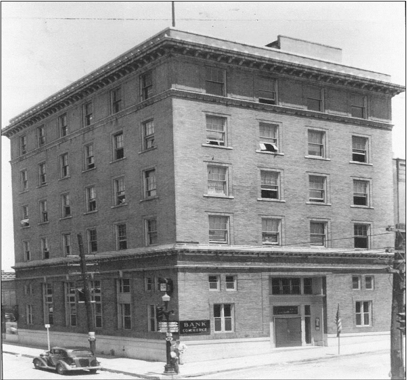
Figure 9. Bank of Commerce Building (#16), circa 1940. The main floor of the bank façade has been modified several times since its construction in 1918. Just before the Skymart was installed, a black granite panel surround had been added to the bank's entrance on Main Street and first floor windows on this façade had been filled in. This is one of several examples in the district that demonstrates façade alterations prior to the installation of the Skymart.
