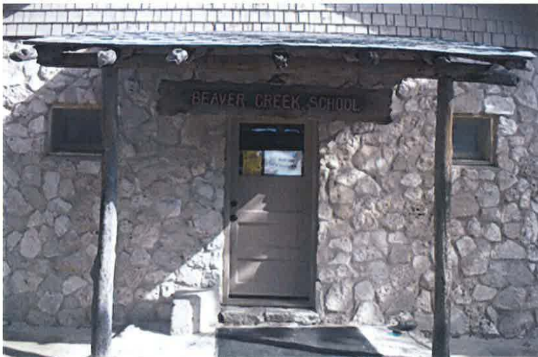
AZ_Yavapai County_Beaver Creek School_0008
