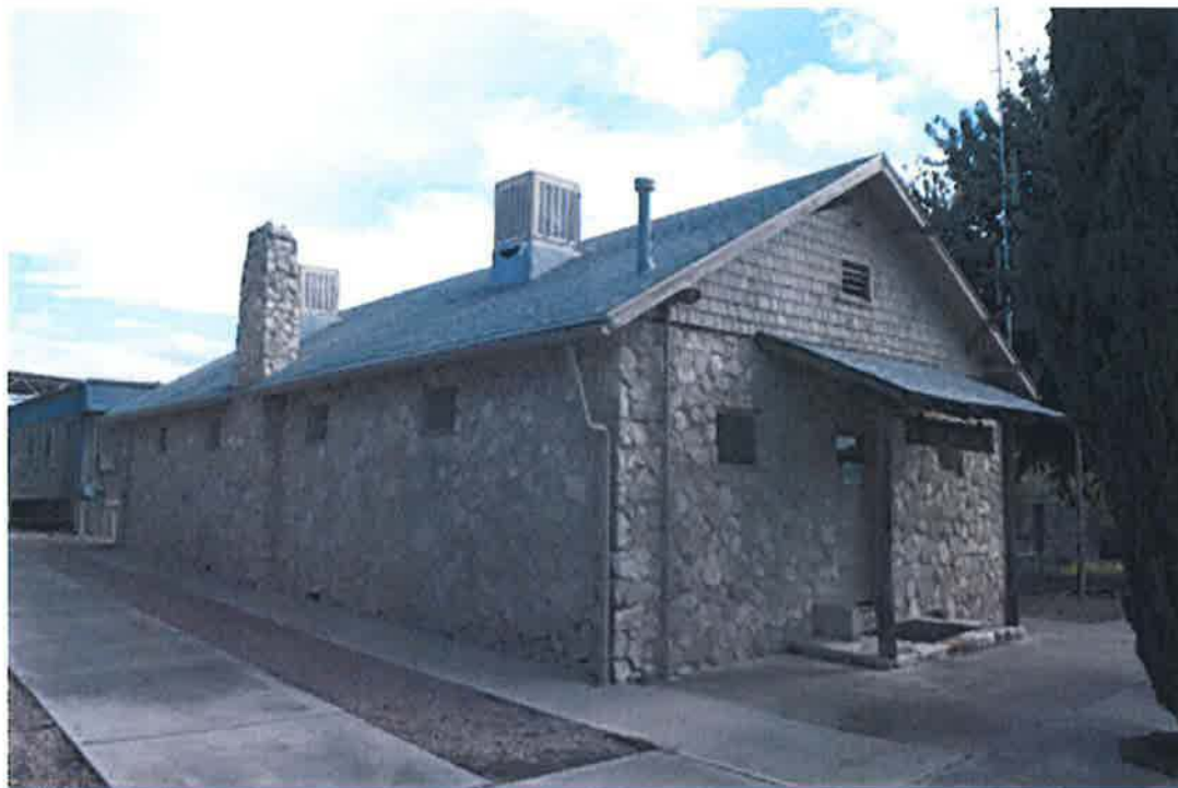
AZ_Yavapai County_Beaver Creek School_0001
