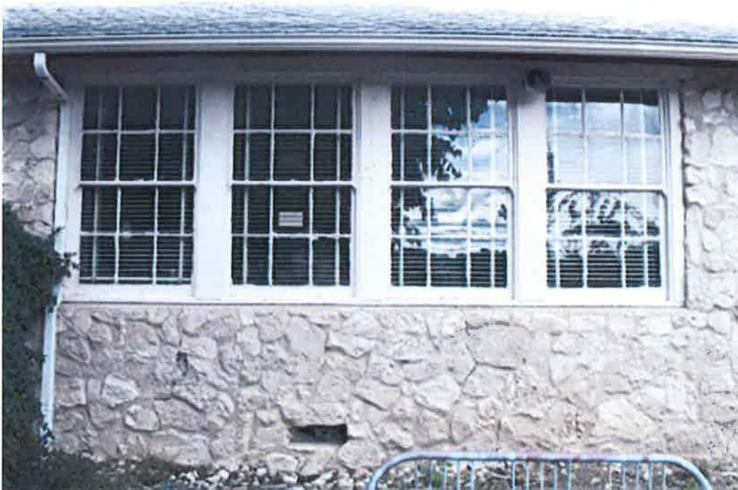
AZ_Yavapai County_Beaver Creek School_0006
