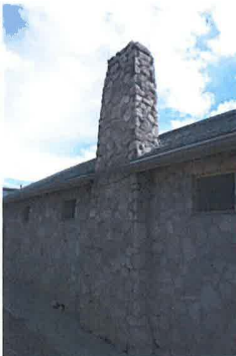
AZ_Yavapai County_Beaver Creek School_0002
