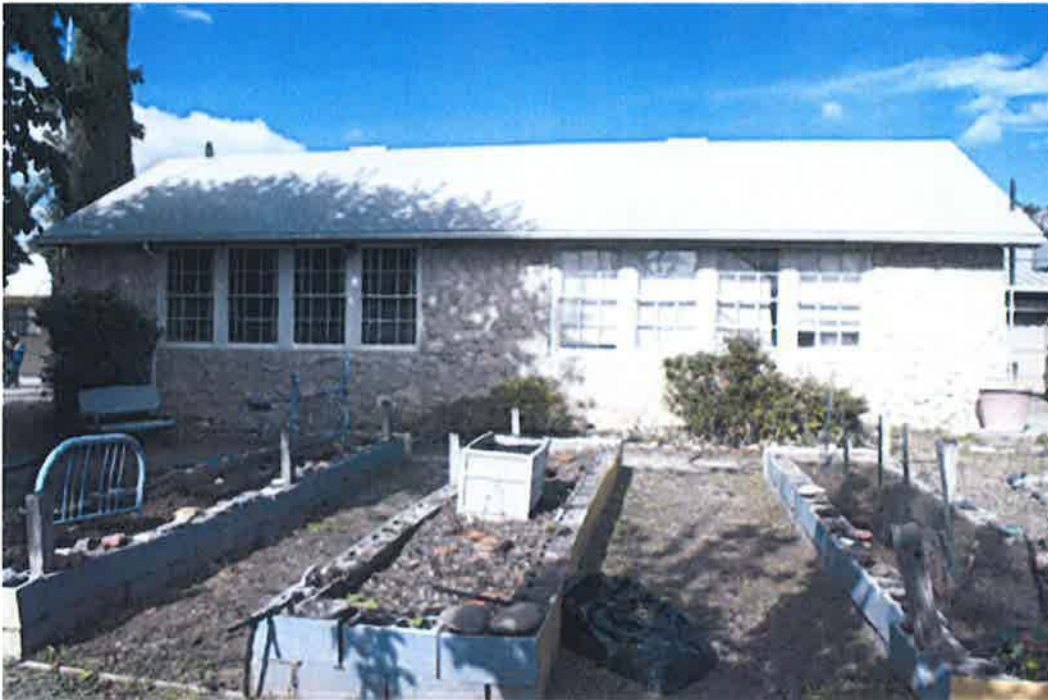
AZ_Yavapai County_Beaver Creek School_0005
