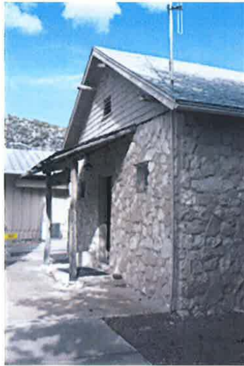
AZ_Yavapai County_Beaver Creek School_0007
