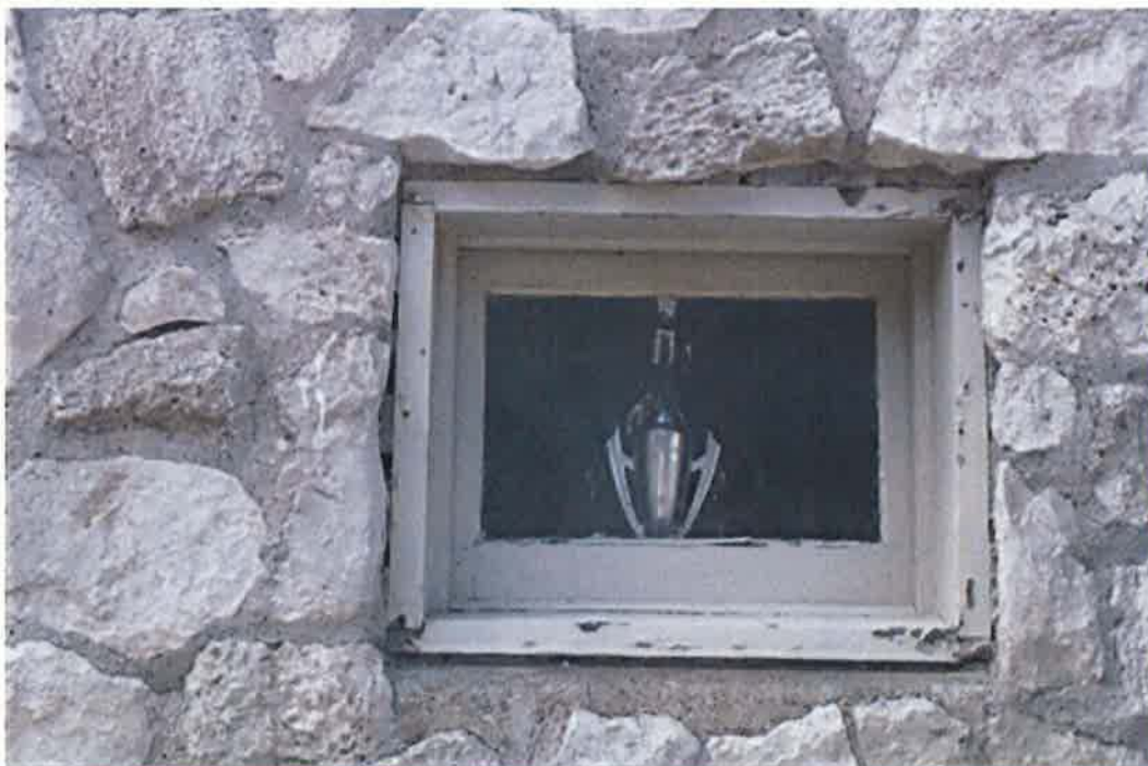
AZ_Yavapai County_Beaver Creek School_0004
