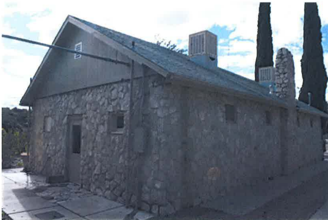
AZ_Yavapai County_Beaver Creek School_0003
