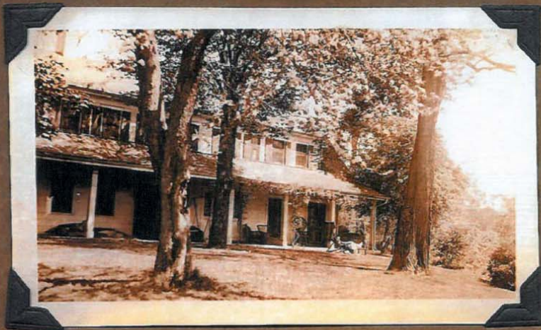
Figure 10: From the top: the front, side and rear views, 1933. Courtesy: Concerned Citizens of Allendale, Inc.
