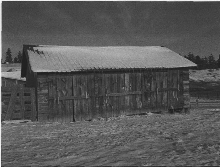
Name: Cheever/Cain Ranch County and State: Powder River County, Montana Photographer: Ella Mae Howard Date of Photograph: 12/4/2009 Location of original negative: State Historic Preservation Office, Helena, MT Description and view of camera: Garage, south elevation. View to north. Photograph Number: 0008
