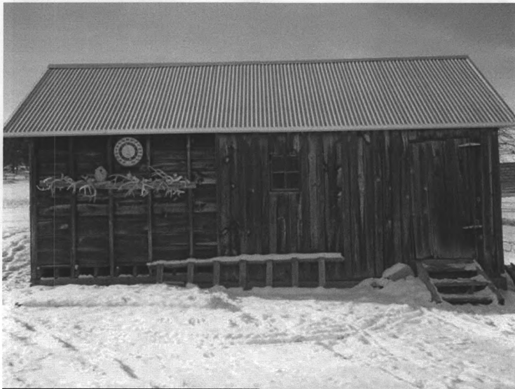
Name: Cheever/Cain Ranch County and State: Powder River County, Montana Photographer: Ella Mae Howard Date of Photograph: 12/4/2009 Location of original negative: State Historic Preservation Office, Helena, MT Description and view of camera: Coal Shed, east elevation. View to west. Photograph Number: 0003
