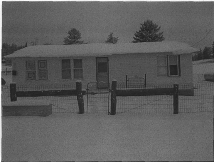
Name: Cheever/Cain Ranch County and State: Powder River County, Montana Photographer: Ella Mae Howard Date of Photograph: 12/4/2009 Location of original negative: State Historic Preservation Office, Helena, MT Description and view of camera: House and surrounding fence, east elevation. View to west. Photograph Number: 0002
