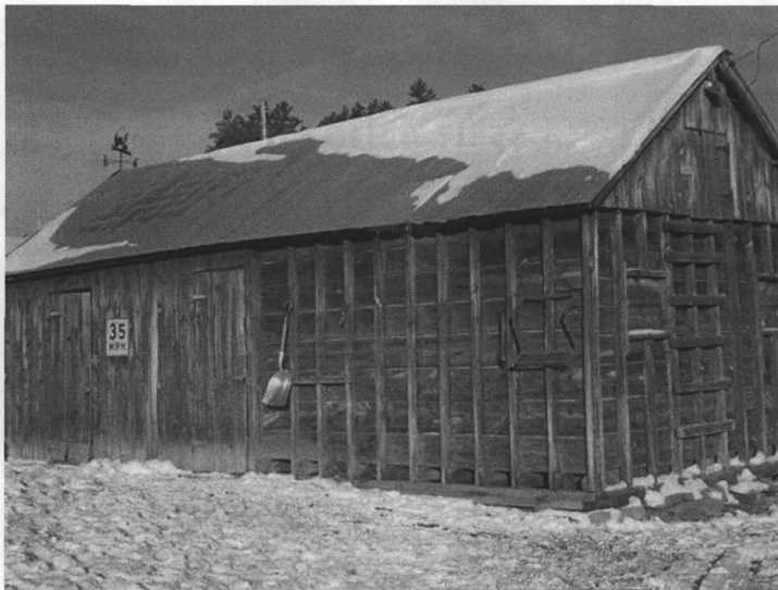
Name: Cheever/Cain Ranch County and State: Powder River County, Montana Photographer: Ella Mae Howard Date of Photograph: 12/4/2009 Location of original negative: State Historic Preservation Office, Helena, MT Description and view of camera: Tool Shop/Granary, south and east elevation. View to northwest. Photograph Number: 0004
