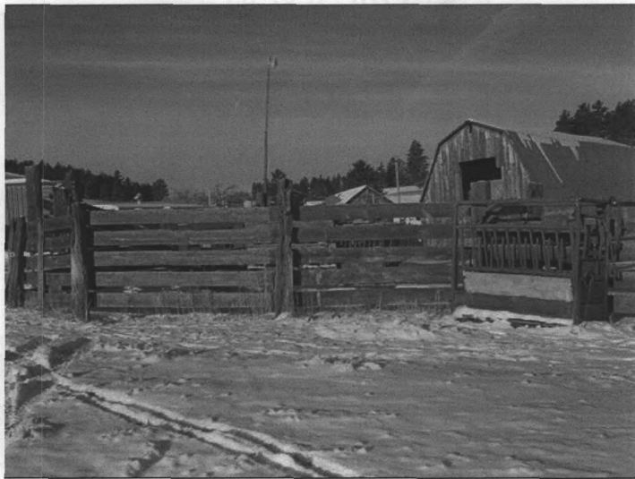
Name: Cheever/Cain Ranch County and State: Powder River County, Montana Photographer: Ella Mae Howard Date of Photograph: 12/4/2009 Location of original negative: State Historic Preservation Office, Helena, MT Description and view of camera: Corrals. View to northwest. Photograph Number: 0011
