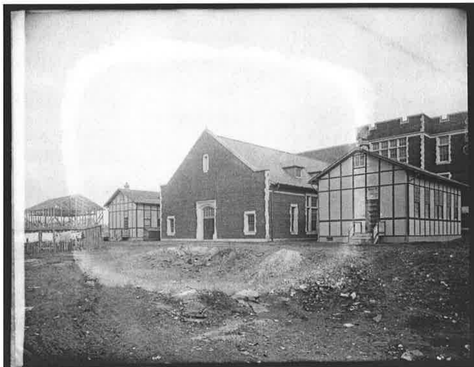
West façade of school showing auditorium and construction of portable classrooms ca. 1919 (Library of Congress, Prints and Photographs Division)
