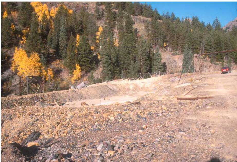
HP 15. 2001 photo of Tailings Impoundment 6, looking west. This area was remediated and covered with waste rock in 2013.
