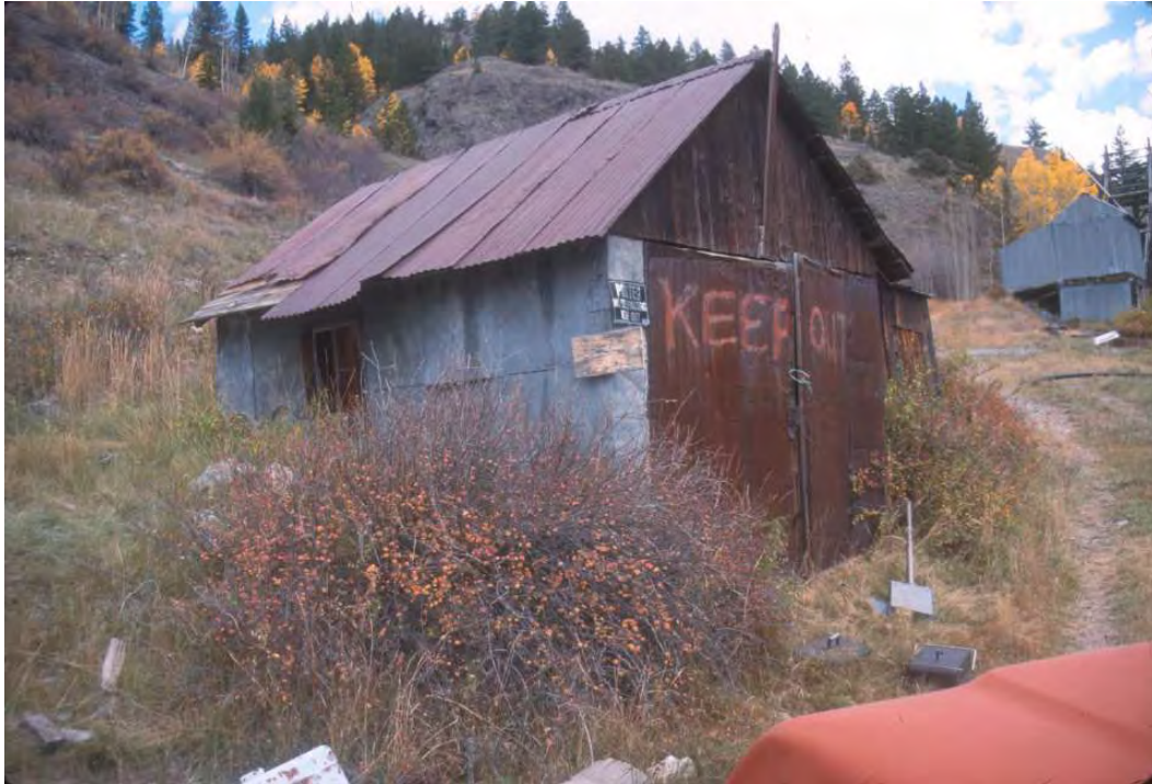
HP 24. 2001 photo of the southwestern and northwestern sides of Building 39, looking east. This building later collapsed and was removed.
