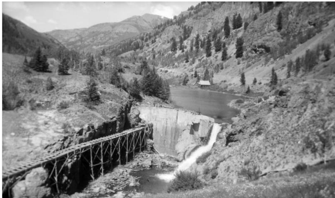
HP 2. The concrete dam (Feature 1) across Henson Creek and the initial part of the flume (Feature 2). Photo taken about 1942 by Muriel Sibell Wolle. DPL photo X-4166
