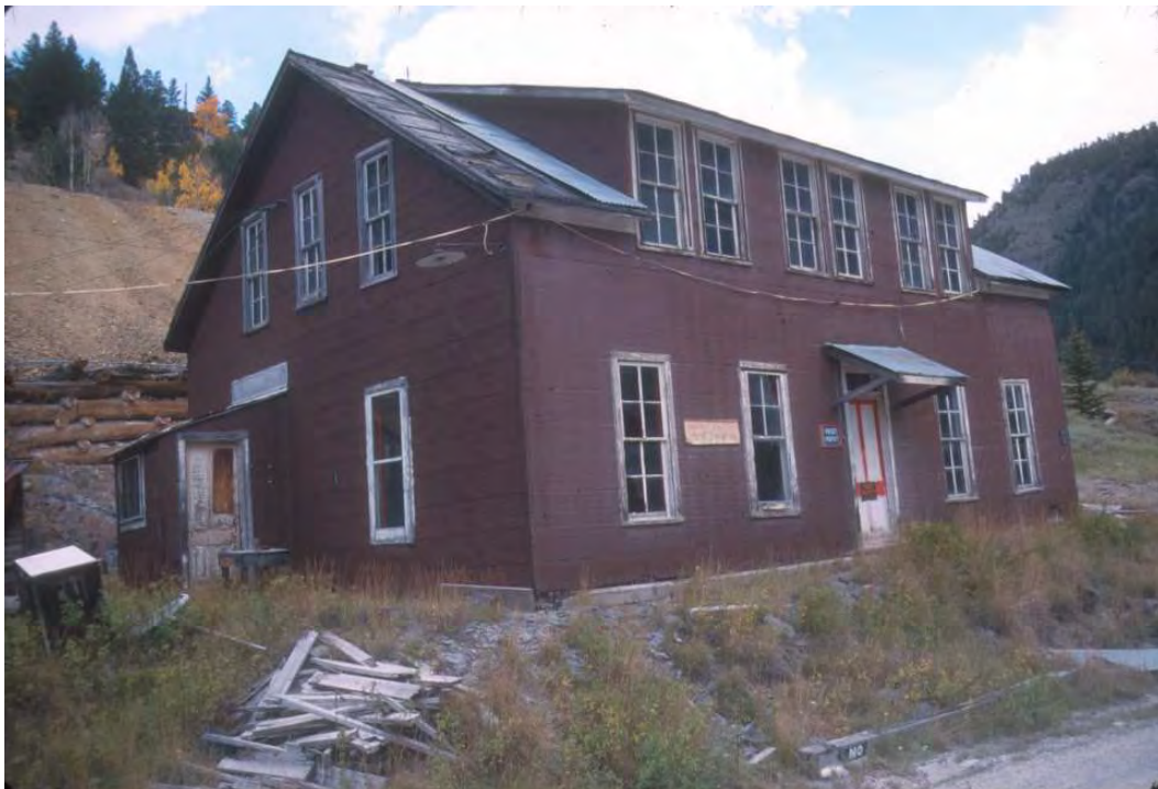
HP 17. 2001 photo of the southwestern and northwestern sides of the boarding house (Building 16), looking east-southeast. Note the original windows and door in place.
