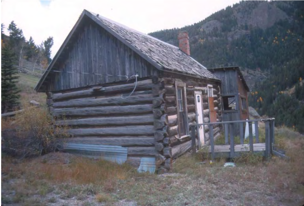
HP 18. Southwestern and northwestern sides of the log cabin residence (Building 17), looking southeast in 2001.
