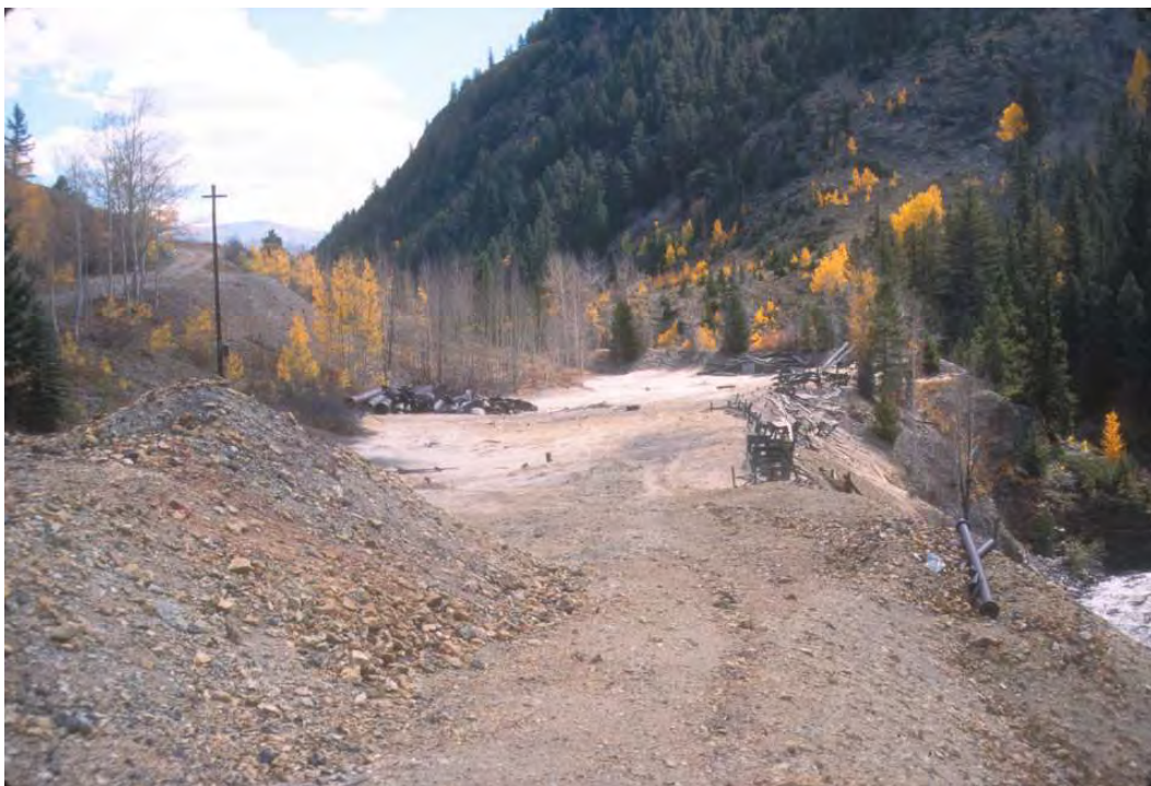
HP 13. 2001 photo of Tailings Impoundment 7 with Henson Creek adjacent to the right. View is to the east.
