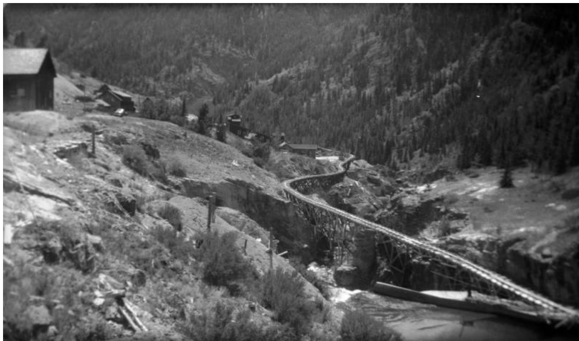
HP 5. The flume (Feature 2) winding southeastward down Henson Creek with the office (Building 9) just above the flume and the mill (Building 6) at center. At the far right is removed Building 36 with the boarding house (Building 16) in the distance. Photo taken in 1942 by Muriel Sibell Wolle. DPL photo X-3474
