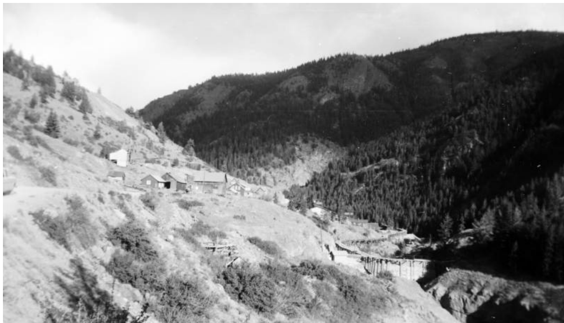
HP 3. Looking southeast at the Henson portion of the Ute-Ulay Mine and Mill. Note the concrete dam across Henson Creek with the gauging station (Building 35) to its left and the flume winding its way to the mill buildings in the distance. In the upper left is the hoist house/transformer house (Building 25). Immediately below it is the removed shed (Building 39) with Buildings 38 and 37 immediately to its right and removed Structure 36 farther right. In the distance can be seen the boarding house (Building 16). Photo taken about 1959 by Muriel Sibell Wolle. DPL photo X-3475.
