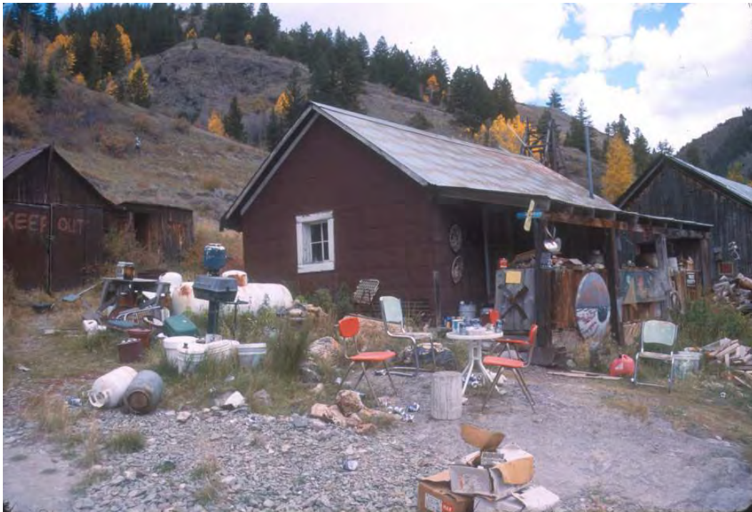
HP 23. 2001 photo of the southwestern and northwestern sides of residence (Building 38), looking east with removed Building 39 to left.
