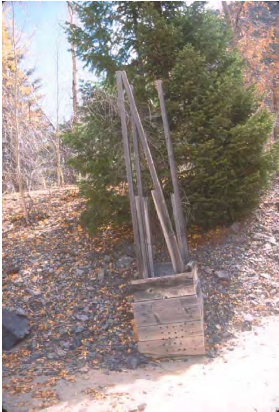
HP 14. Cribbed water drainage box (Feature 4) on east end of Tailings Impoundment 7 as it appeared in 2001, looking east-southeast. This was removed during mill tailings remediation in 2013.
