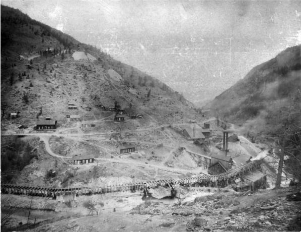
HP 1. Ute-Ulay Mine and Mill in the 1880s. See Figure 1 for explanation of buildings that still exist. Photo taken between 1883-89 by Frank E. Dean. DPL photo X-61914.
