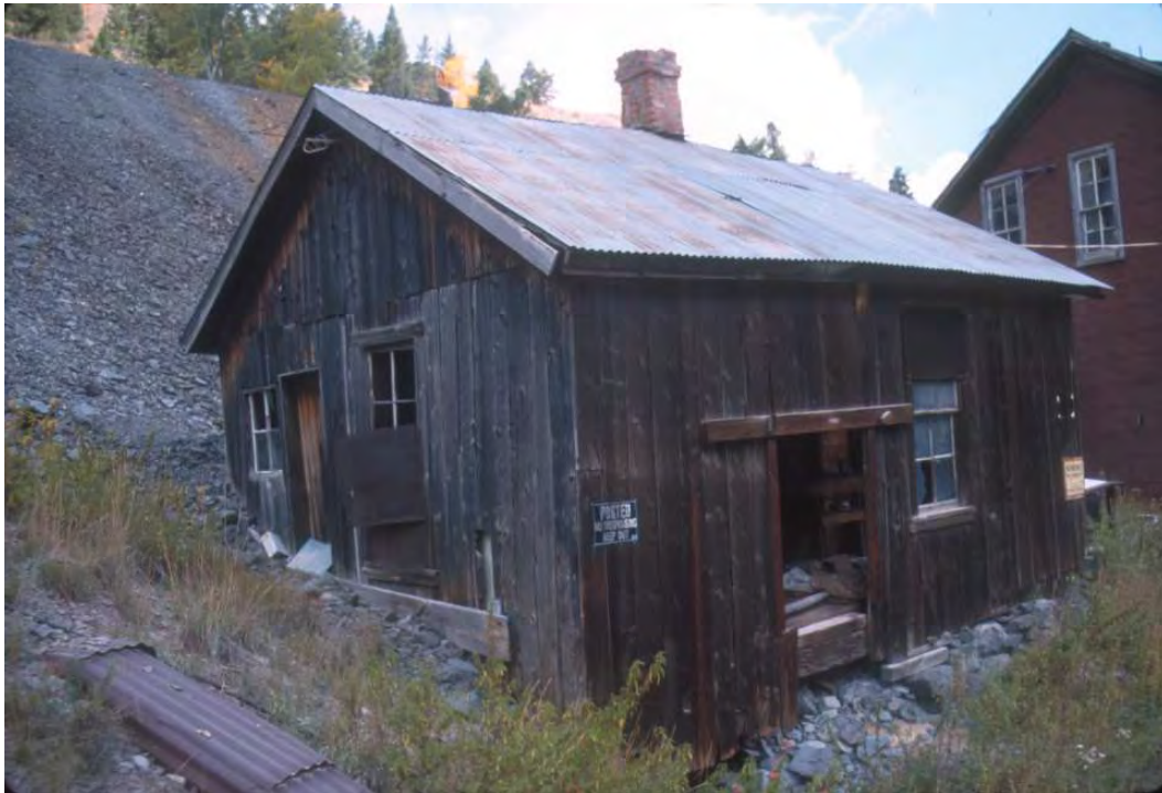
HP 16. 2001 photo of the southwestern and northwestern sides of Building 15, looking east.
