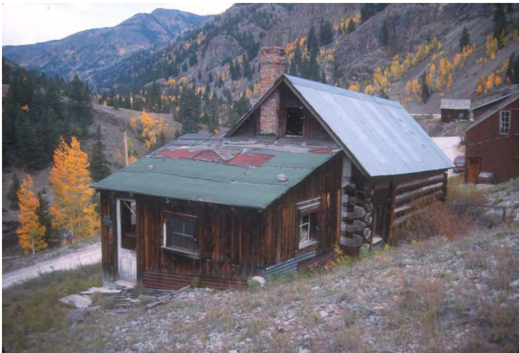
HP 19. Southeastern and northeastern sides of the log cabin residence (Building 17), looking northwest.
