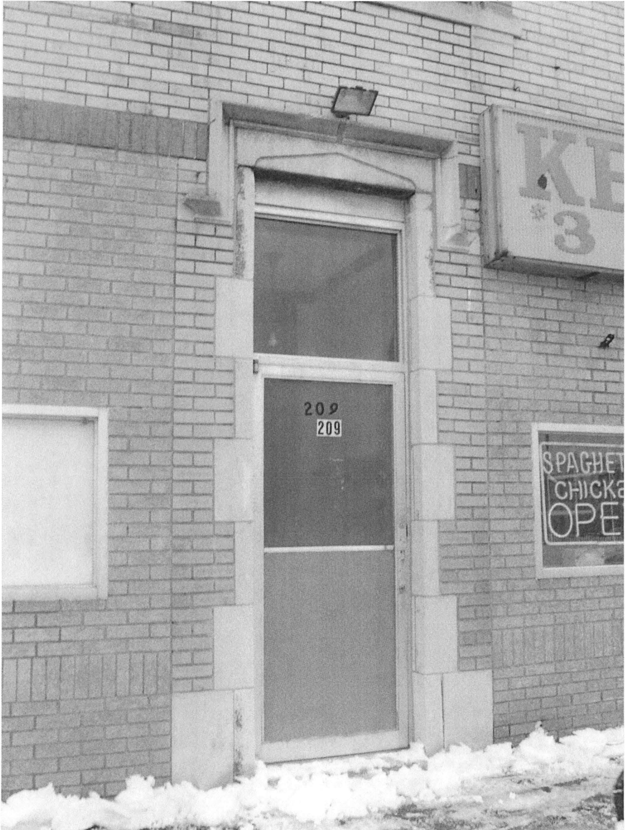
East (front) elevation of building from Garden Street, showing east entry detail. Camera facing northwest. Photograph 2 of 11
