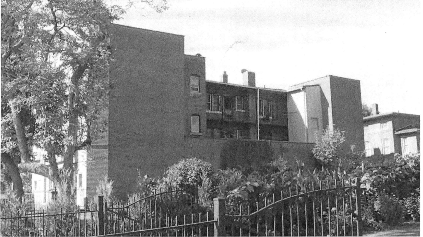
North (side) elevation of building from Garden Street, showing rear porch and stairwell details. Camera facing southwest. Photograph 6 of 11
