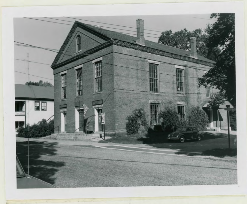
Old Town Hall, 1358 South (Front) Elevation and East Side
