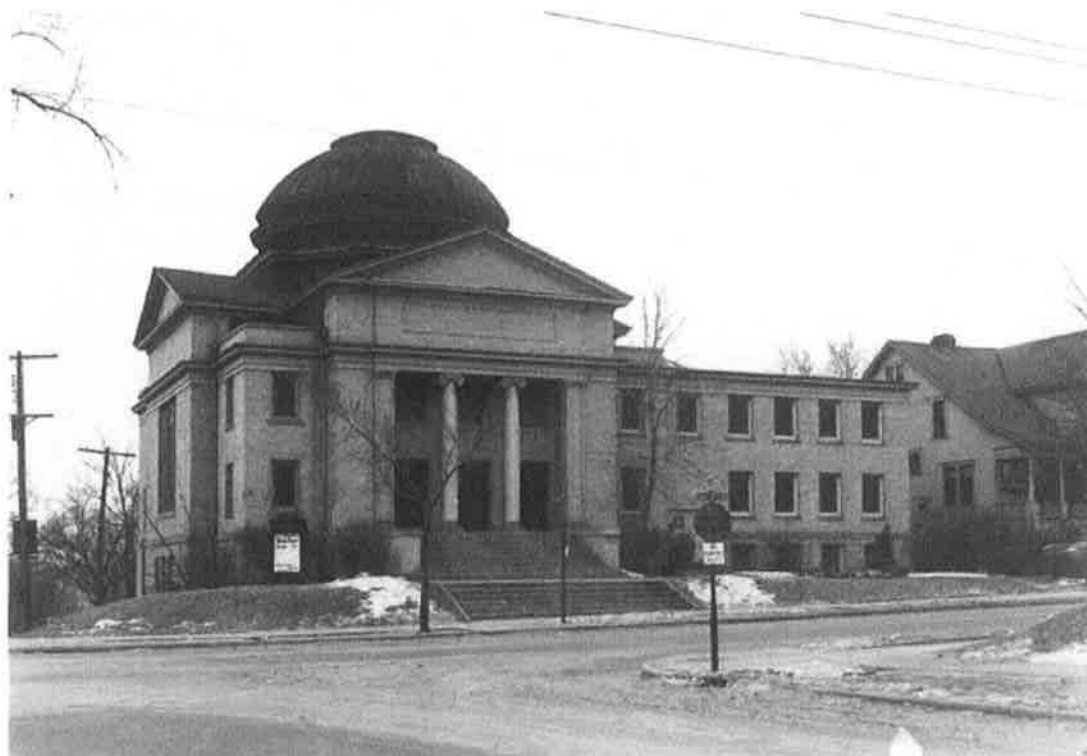
Figure 1. Lake Harriet Methodist Episcopal Church, ca. 1920 -1930. Minneapolis Photo Collection, Hennepin County Library.
