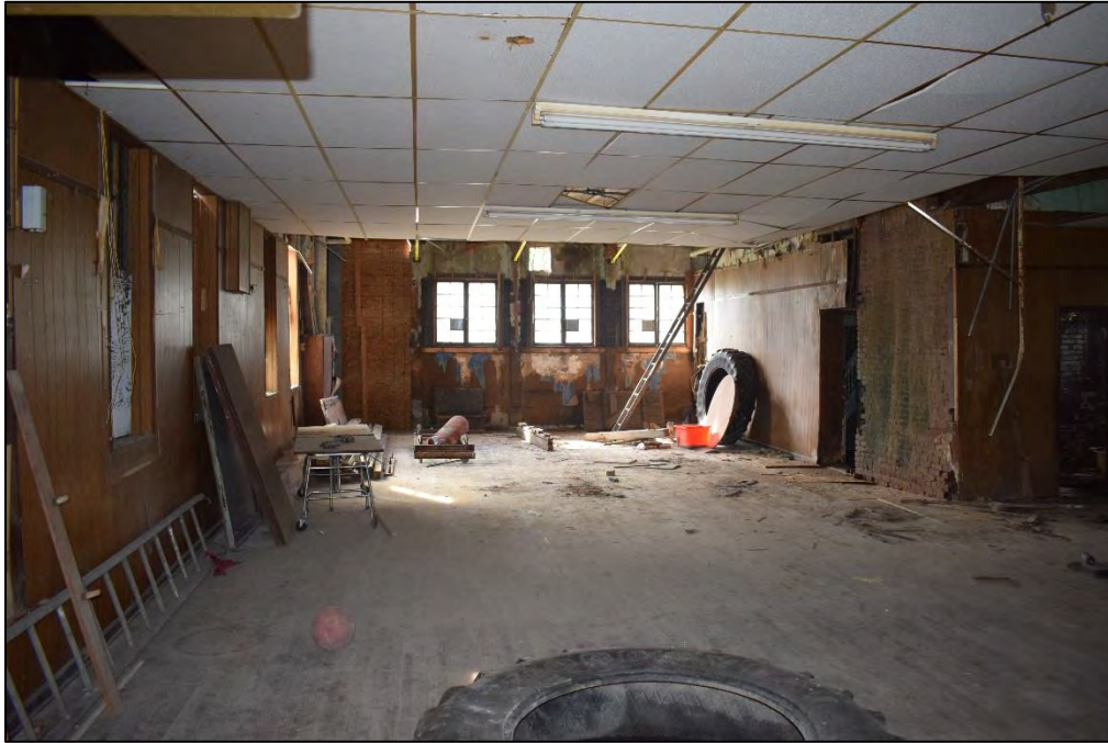
View of the main room on the first floor, facing west.
