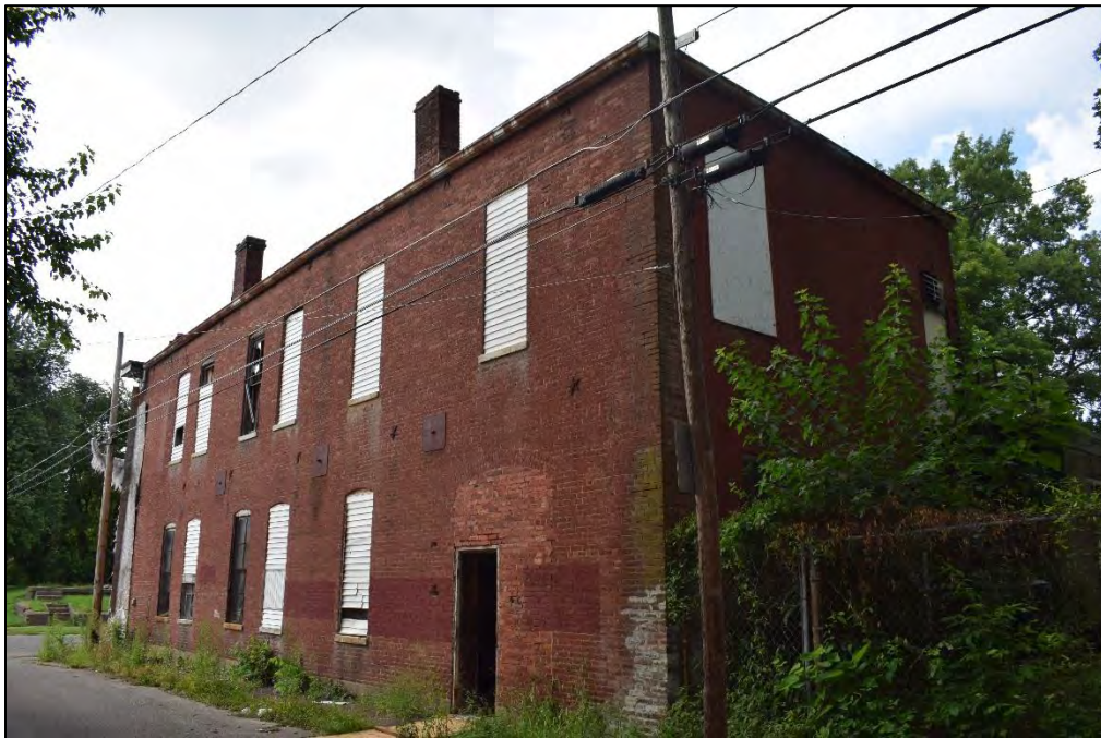
South and east elevations of Shafer's Hall, facing northwest.
