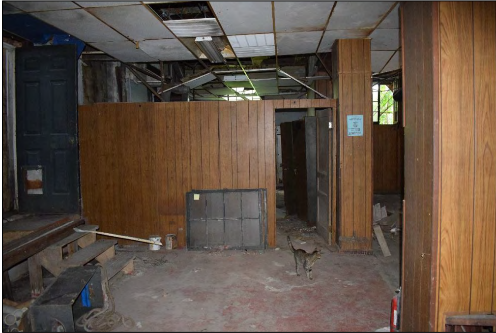
Concrete block addition, facing east.
