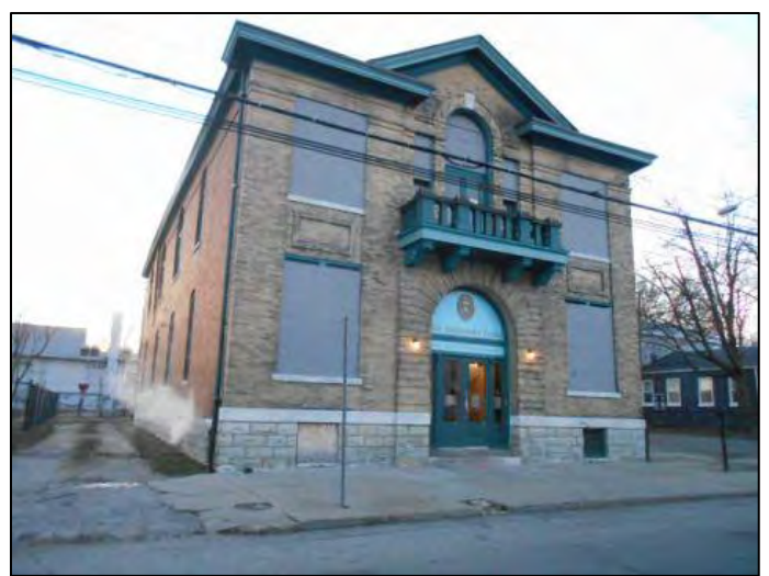
Lewis Hall (Jefferson County PVA)
