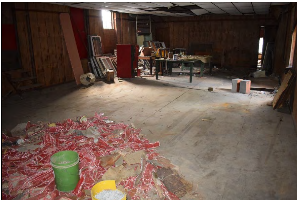
Large room on the second floor, facing west.
