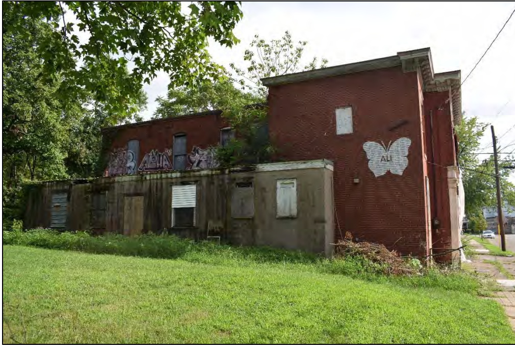
North elevation of Shafer's Hall showing the two additions, facing south.
