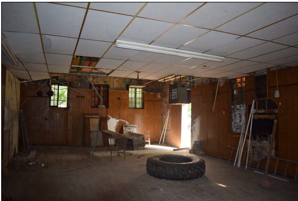
View of the main room on the first floor, facing east.
