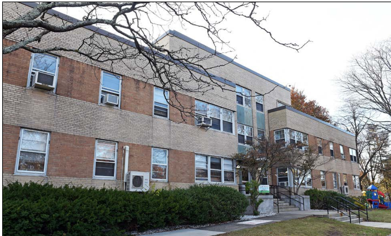
Figure 7. Perspective view of the west elevation of Building #2, November 2017 (VA).
