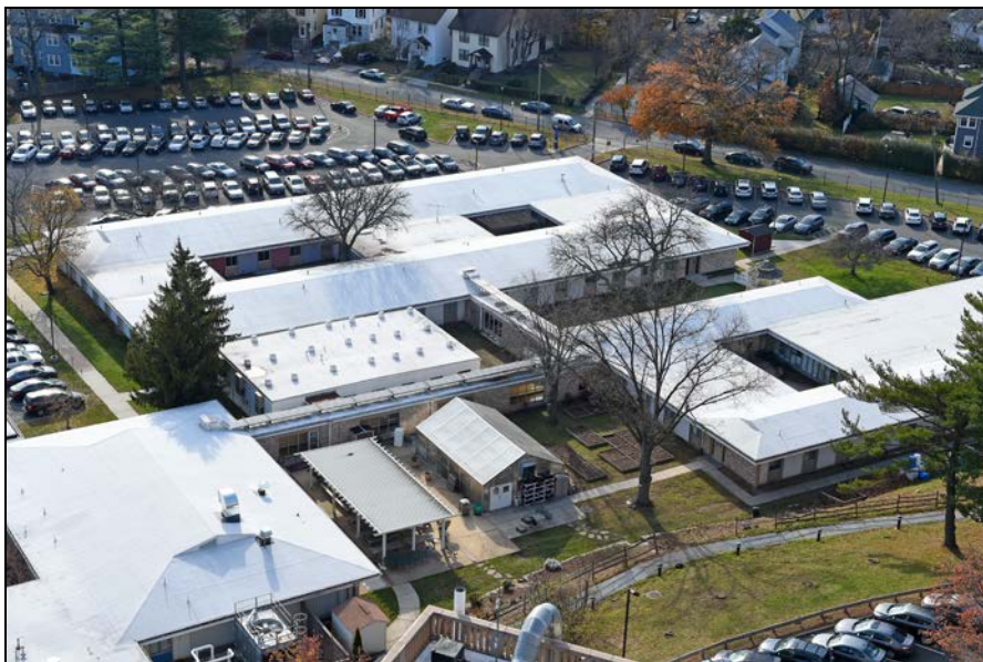
Figure 16. Bird's-eye view of Building #16 (center), Building #17 (right), and Building #15 (left), 2017 (VA).
