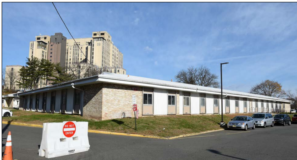
Figure 18. Perspective view of Building #18, November 2017 (VA).
