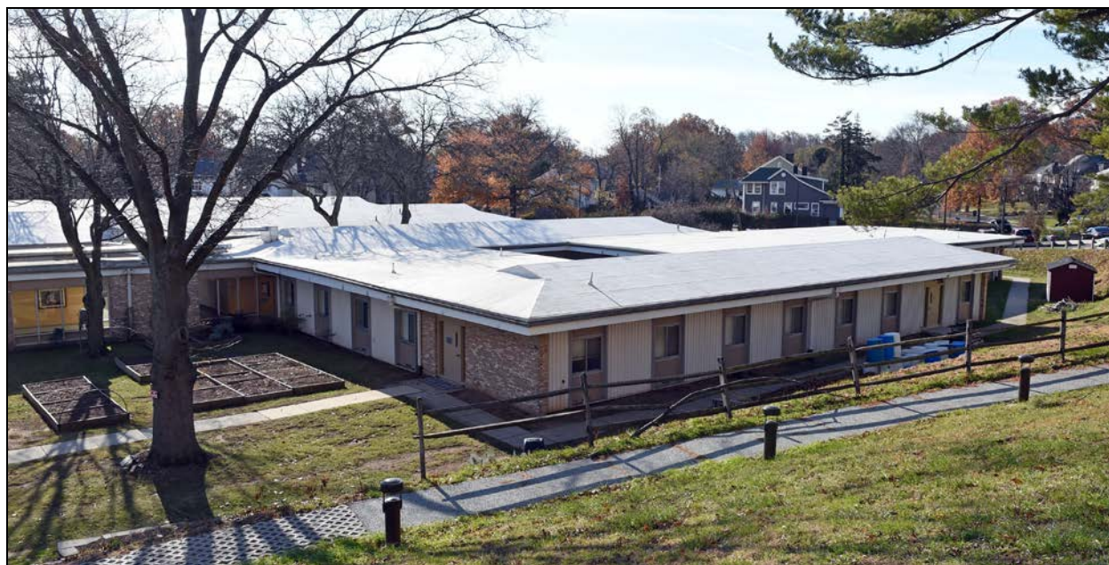
Figure 17. General view looking to Building #17, November 2017 (VA).
