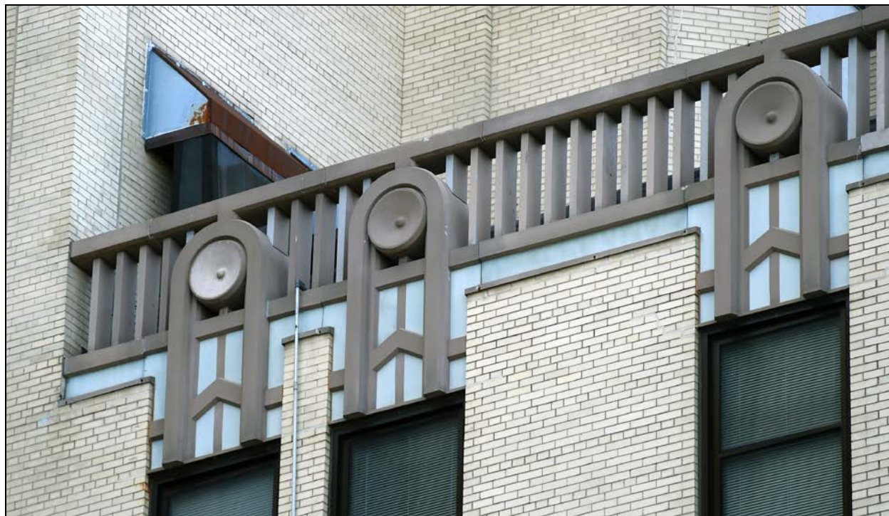
Figure 6. Detail of the roof, November 2017 (VA).
