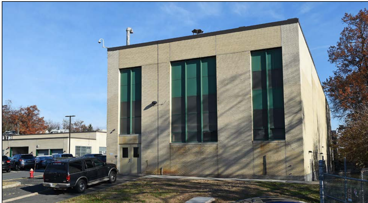
Figure 12. View looking to the southeast elevation with pedestrian entrance, November 2017 (VA).
