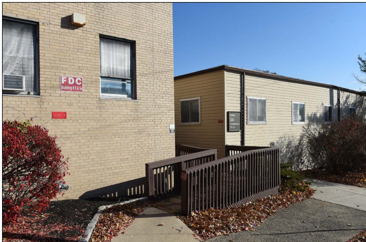
Figure 10. (above) General view of Building #5 and Building #5A to show the buildings' spatial relationship and close view of the connector between the two buildings, November 2017 (VA).
