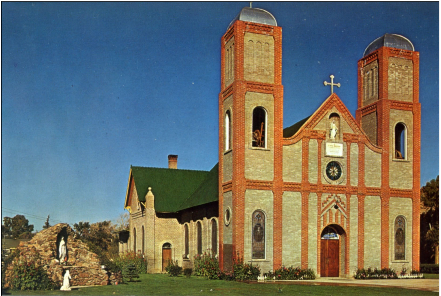
Figure 10. In 1948 the adobe towers and front were removed. The building was extended eastward one bay and the present concrete brick twin towers with aluminum domes constructed. The Lourdes Grotto at left was created in 1954. Courtesy of Thomas H. and R. Laurie Simmons, Our Lady of Guadalupe , ca. late 1950s-early 1960s, historic postcard collection, Denver, Colorado.
