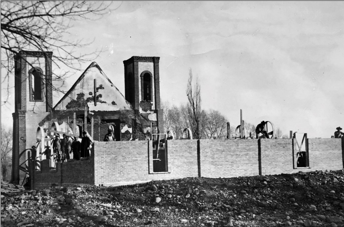
Figure 5. Following a devastating February 1926 fire that spared only the adobe towers and front wall, the church was rebuilt in 1926-27. Courtesy of Stephen H. Hart Library and Research Center, History Colorado, Denver, Colorado.
