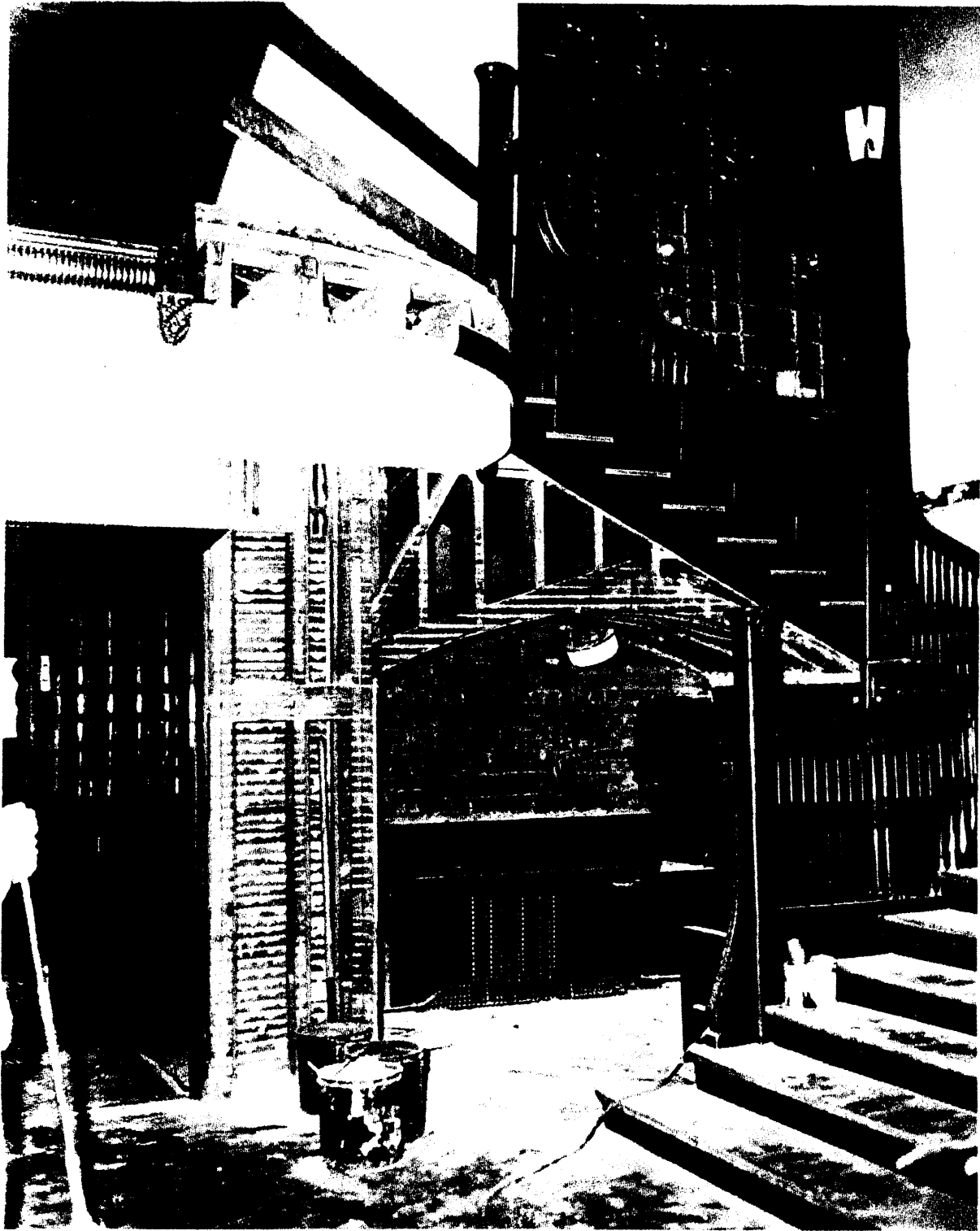
Figure 6. The stair hall during removal of the staircase in the 1950s. The original exterior doors are still visible at the left.
