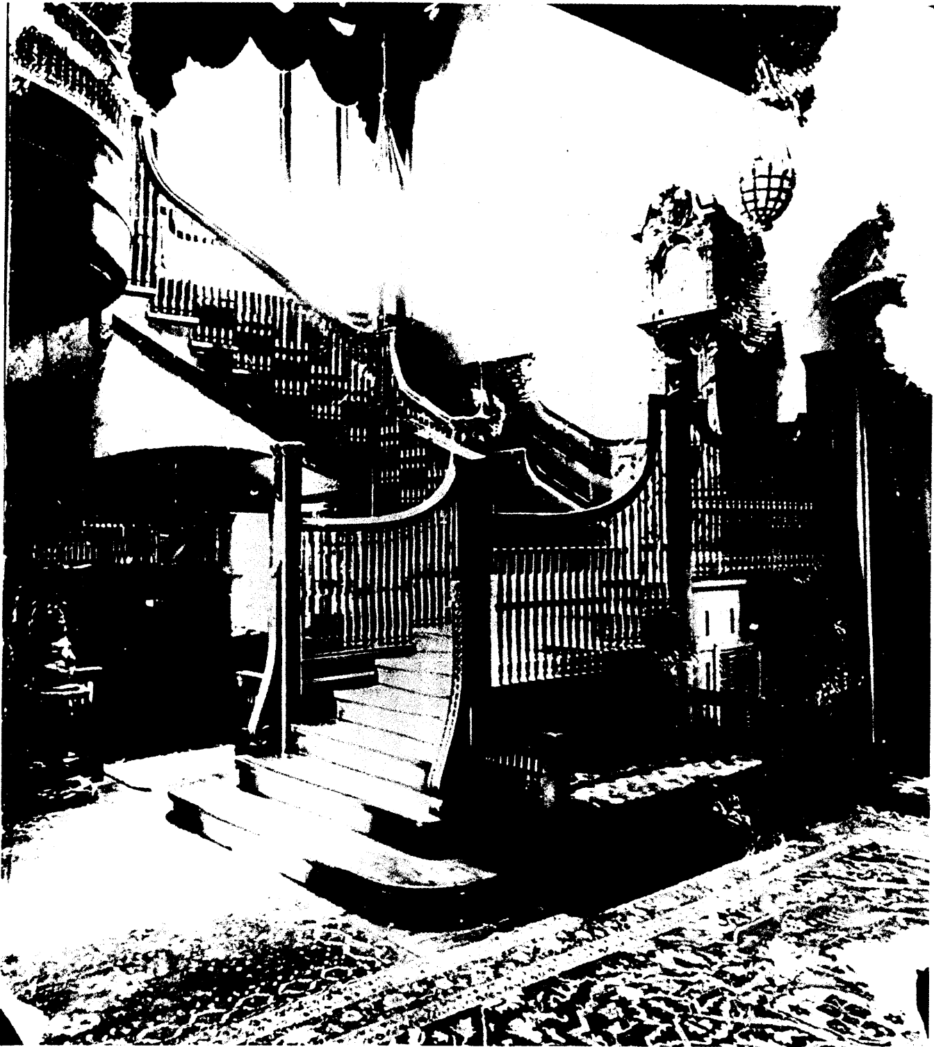
Figure. 5. The stair hall before removal of the original staircase. The spindles on the railing match those to be found on many of the interior shutters. The arched ceiling is visible over the inglenook against the south wall.
