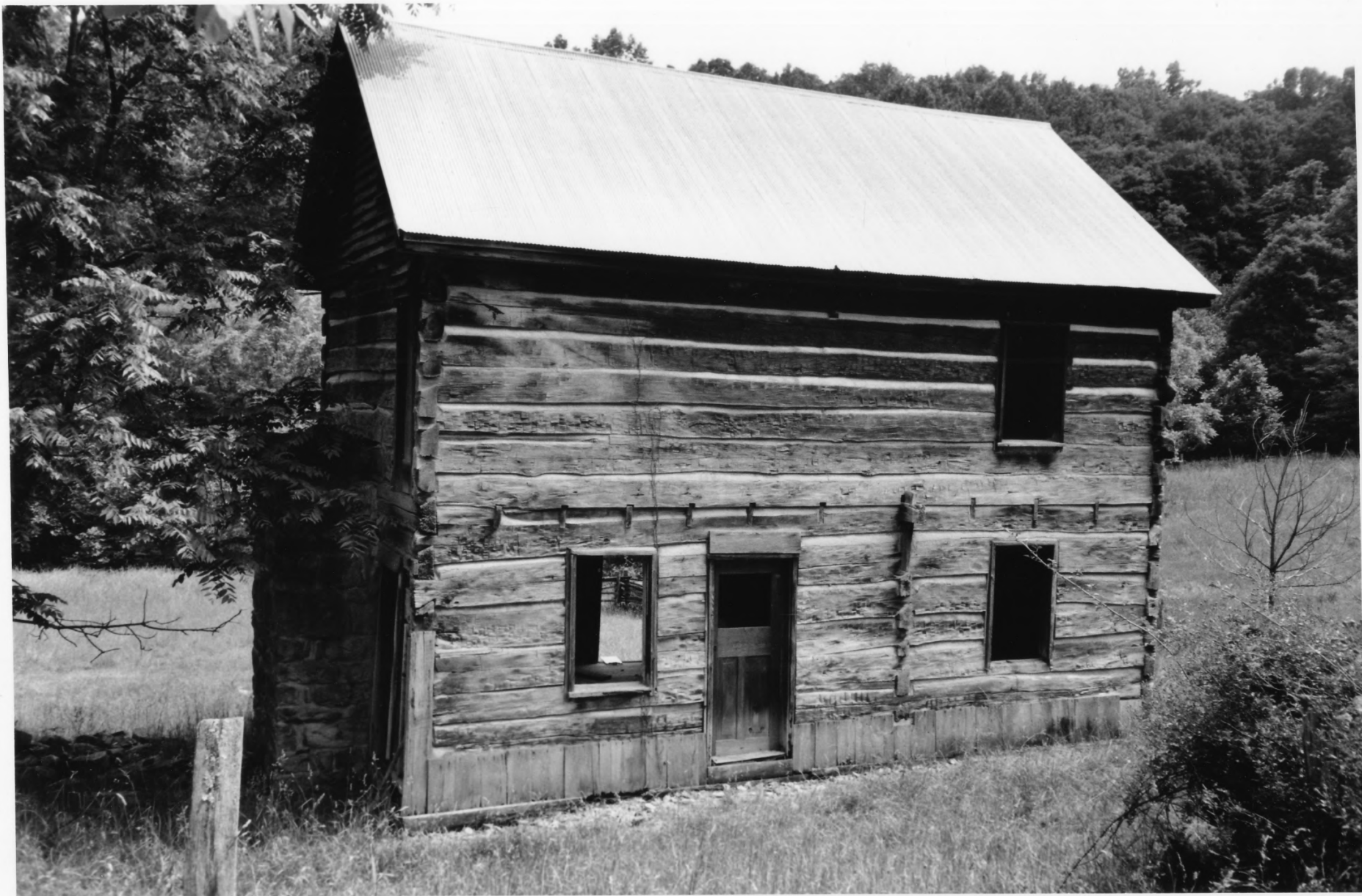
ROHRBAUGH CABIN GRANT CO. WY No. 5
