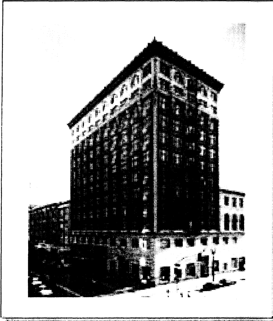
The Brockman Building and New York Cloak & Suit House (Annex) before 2006-2008 rehabilitation. Date unknown.
