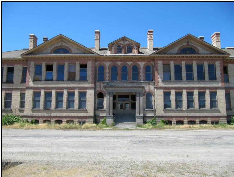
3 of 30 WA_Spokane County_McKinley School_0003.tiff East façade
