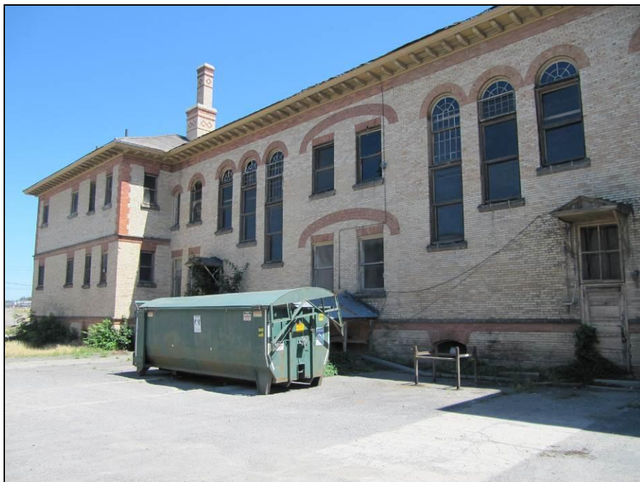
9 of 30 WA_Spokane County_McKinley School_0009.tiff Portion of West/ rear facade, northern half
