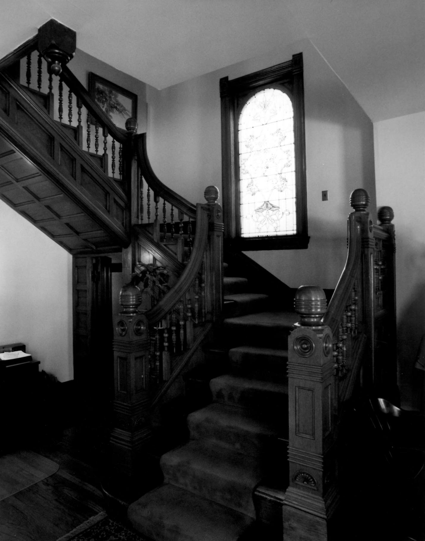
Staircase with stained glass window on second-run of stairway. Detail of newel posts, turned spindles and chamfered under-wall on their run of stairs. Pendant drop at ceiling.
