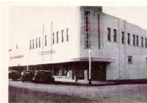
Figure 6: Federated Department Store, 101 S. Dallas Street (center) and Ben Franklin Store, 107 S. Dallas Street (left), Ennis, Texas, c. 1945. This photograph reveals both buildings had received a stucco finish by this date. The Cicerone (Ennis High School Yearbook, 1945).
