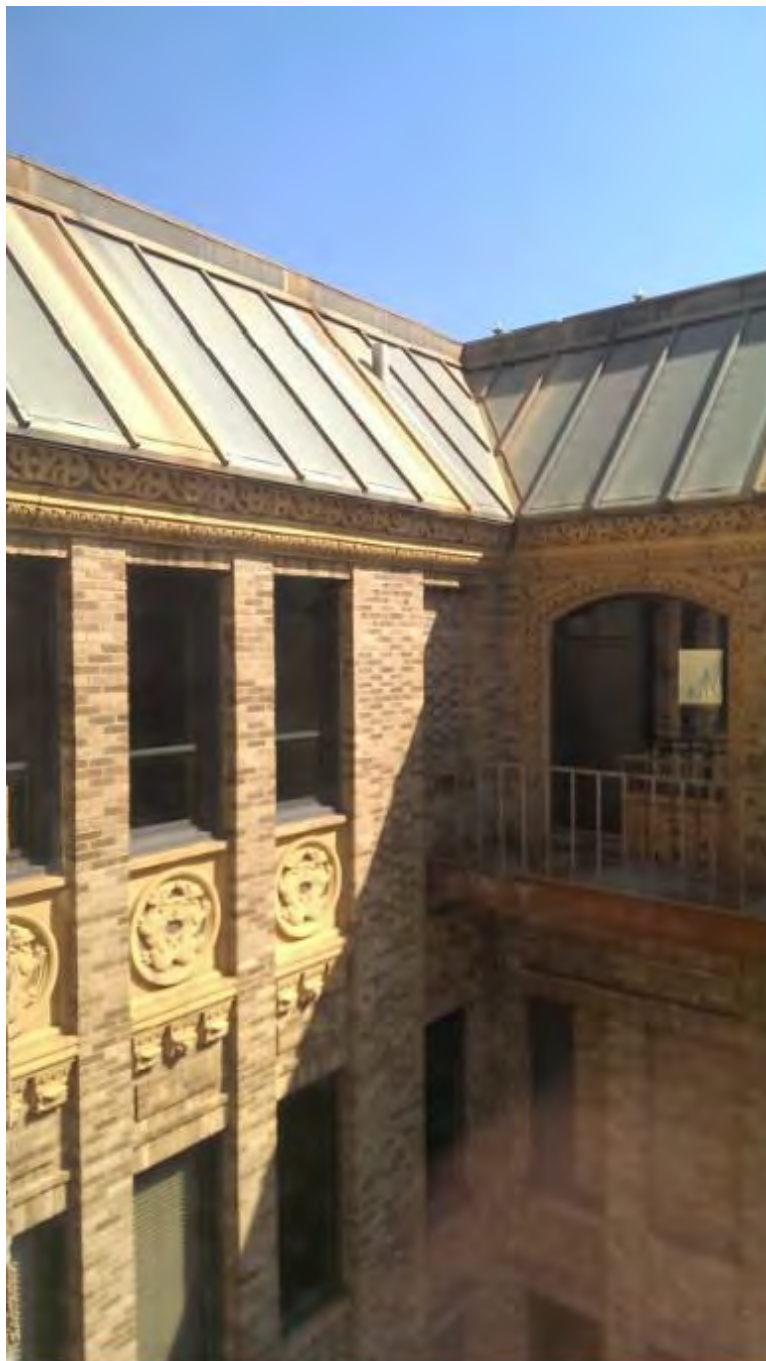
Photo 13: Exterior view of 21 st floor typical terra cotta detailing and copper roof Camera facing east Date: 2015
