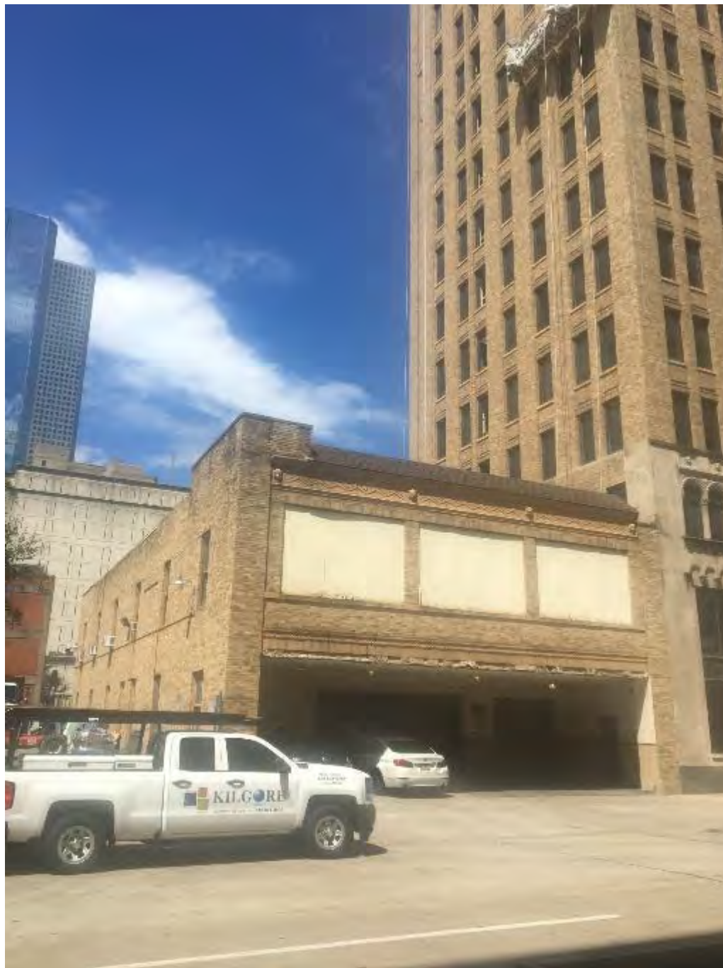
Photo 4: East elevation of attached 2-level garage Camera facing northwest Date: 2018
