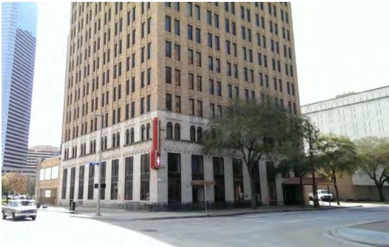
Photo 9: North (primary) and east elevations Camera facing southwest Date: 2015
