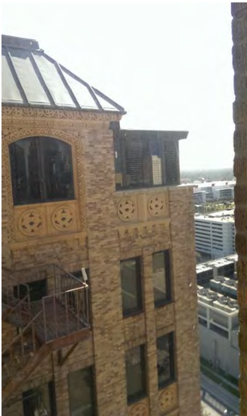
Photo 12: Exterior view of 21 st floor typical terra cotta detailing and copper roof Camera facing south Date: 2015
