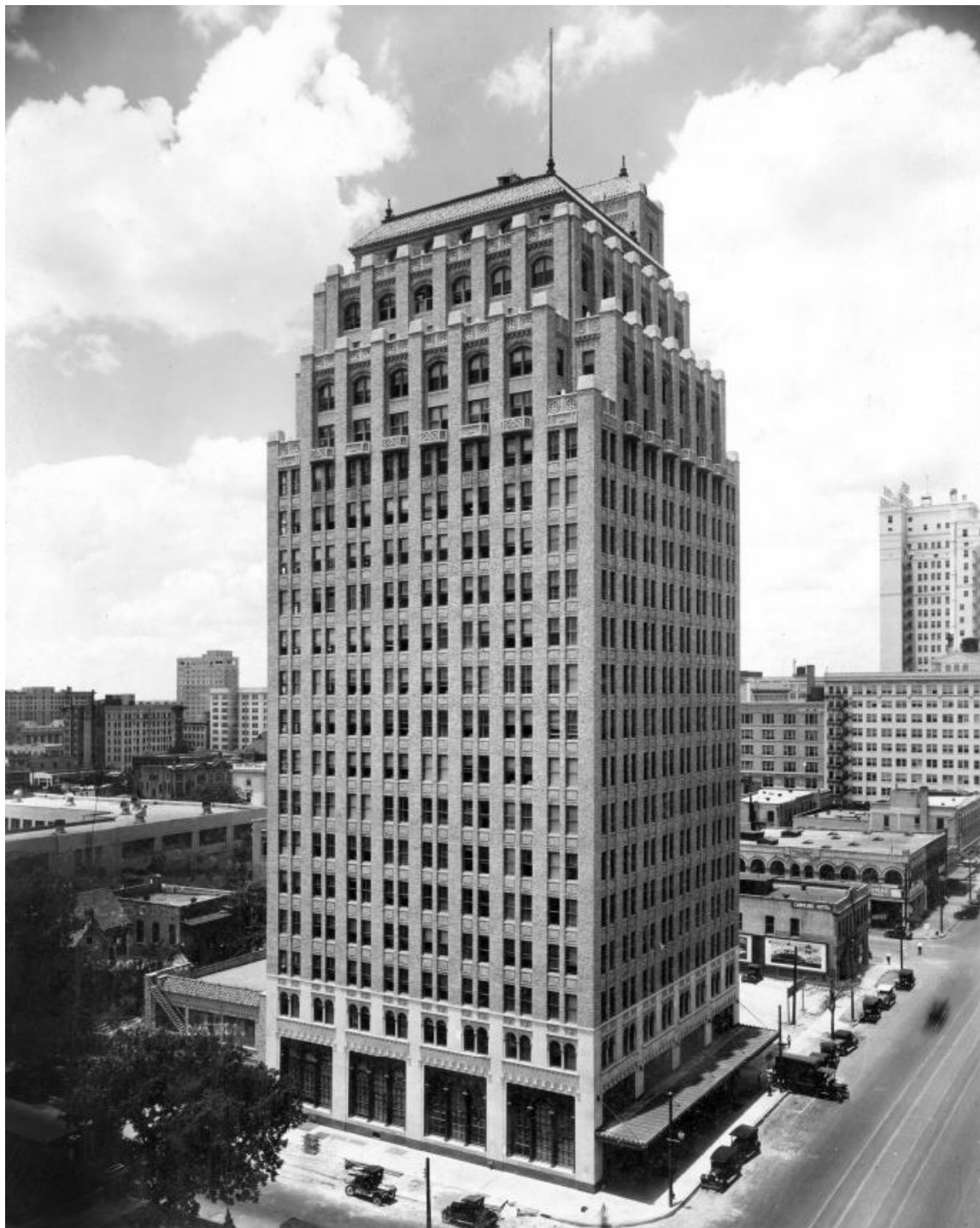
Figure 2: Historic photo, 1928, camera facing west; Courtesy of Houston Metropolitan Research Center, Houston Public Library.
