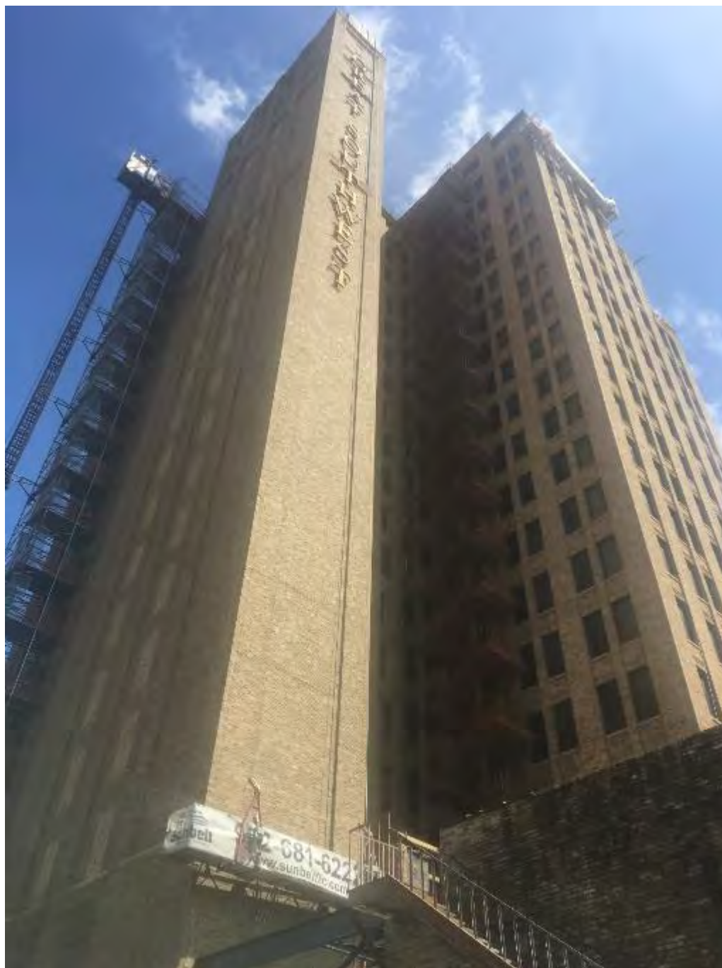
Photo 7: West and south elevations Camera facing northeast Date: 2018
