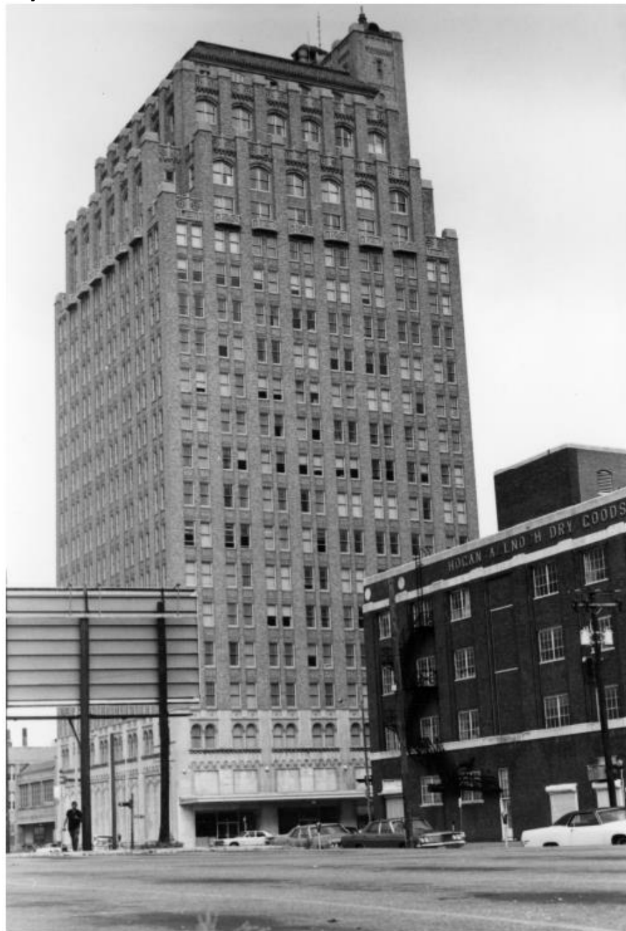
Figure 6: Petroleum Building, 1972, camera facing west; Courtesy of Houston Metropolitan Research Center, Houston Public Library.
