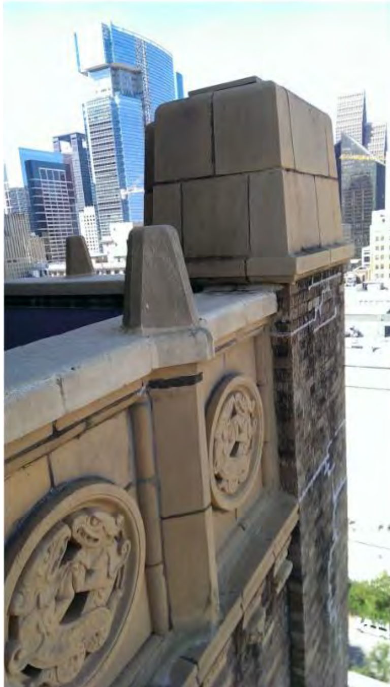
Photo 18: Exterior view of typical terra cotta detailing at parapet Camera facing north Date: 2015
