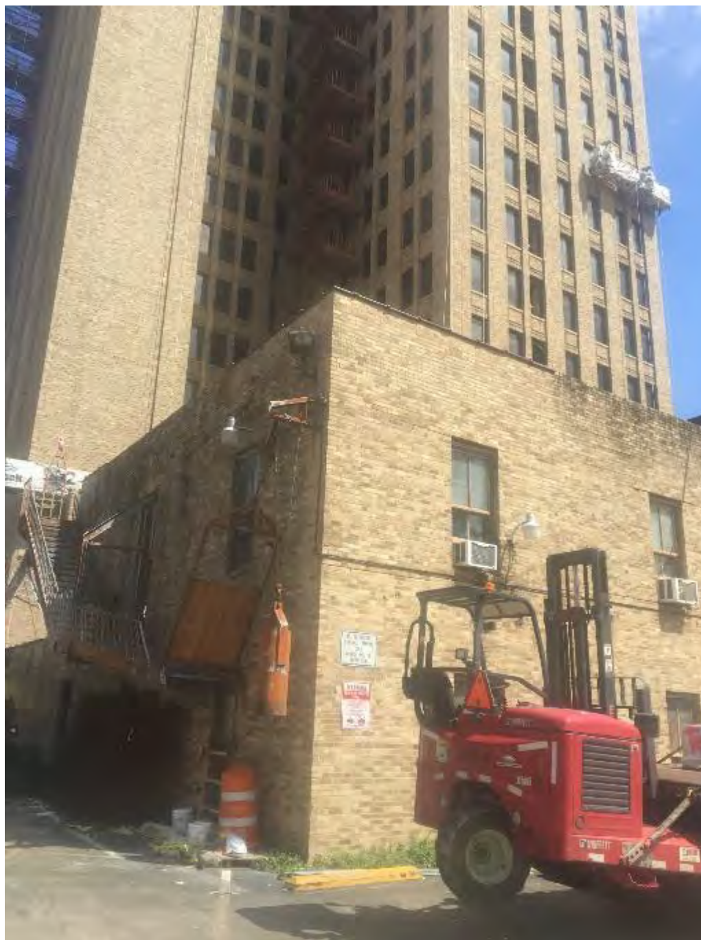
Photo 8: West and south elevations of parking garage Camera facing northeast Date: 2018
