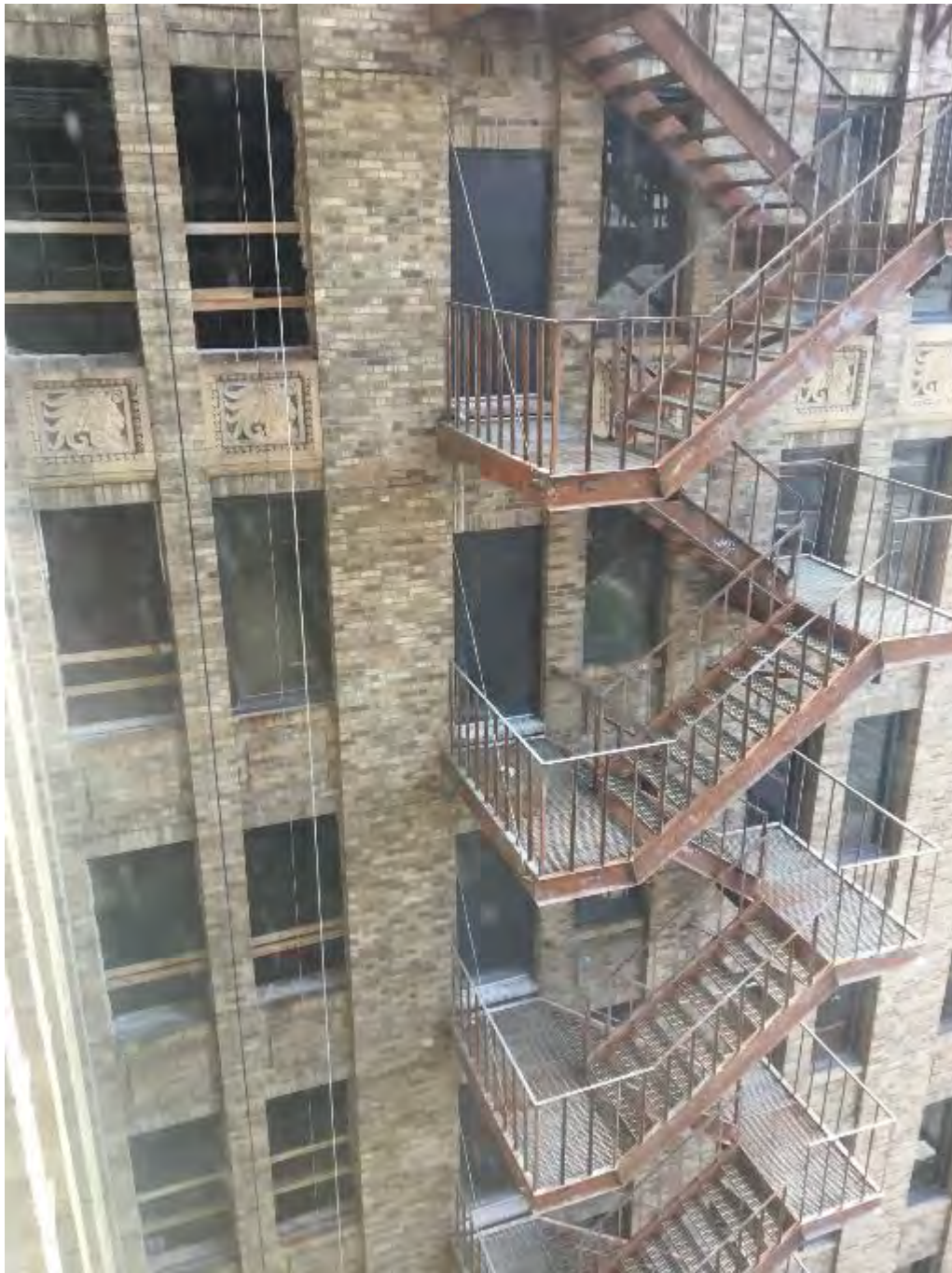
Photo 14: Exterior view of metal fire escape stair Camera facing southeast Date: 2018
