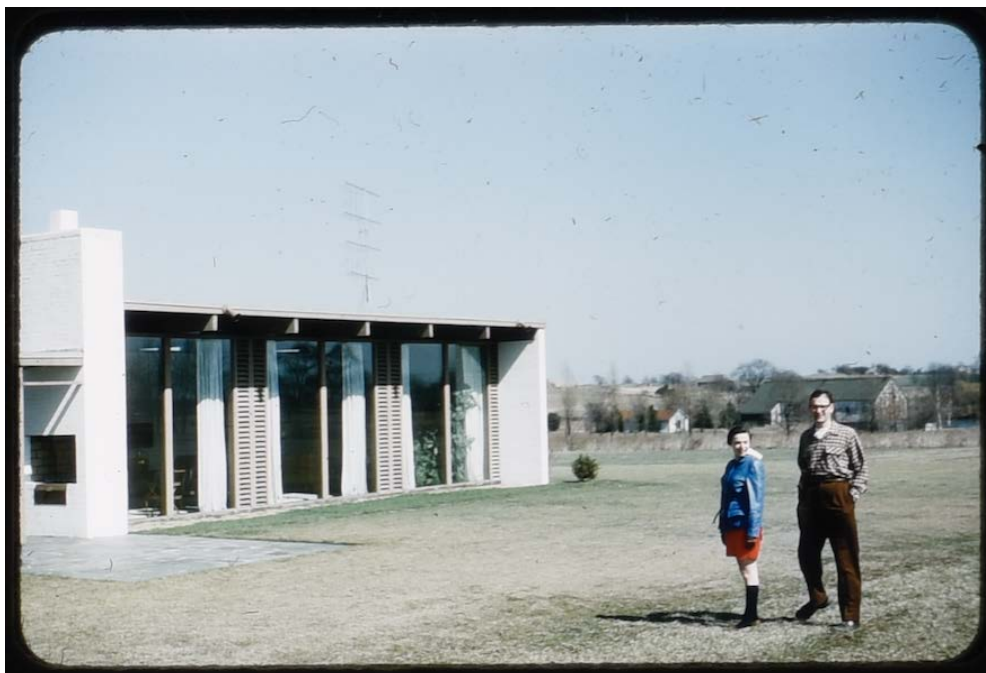
FIGURE 15: Lavin House, south elevation detail, with Audrey and Carl Lavin, 1955. Source: Wisconsin Historical Society Archives.
