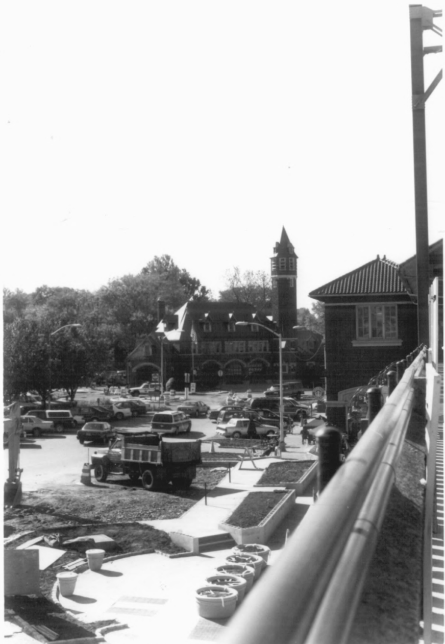
SO. ORANGE FIRE DEPT., SOUTH ORANGE, NJ PHOTO 2 of 12
