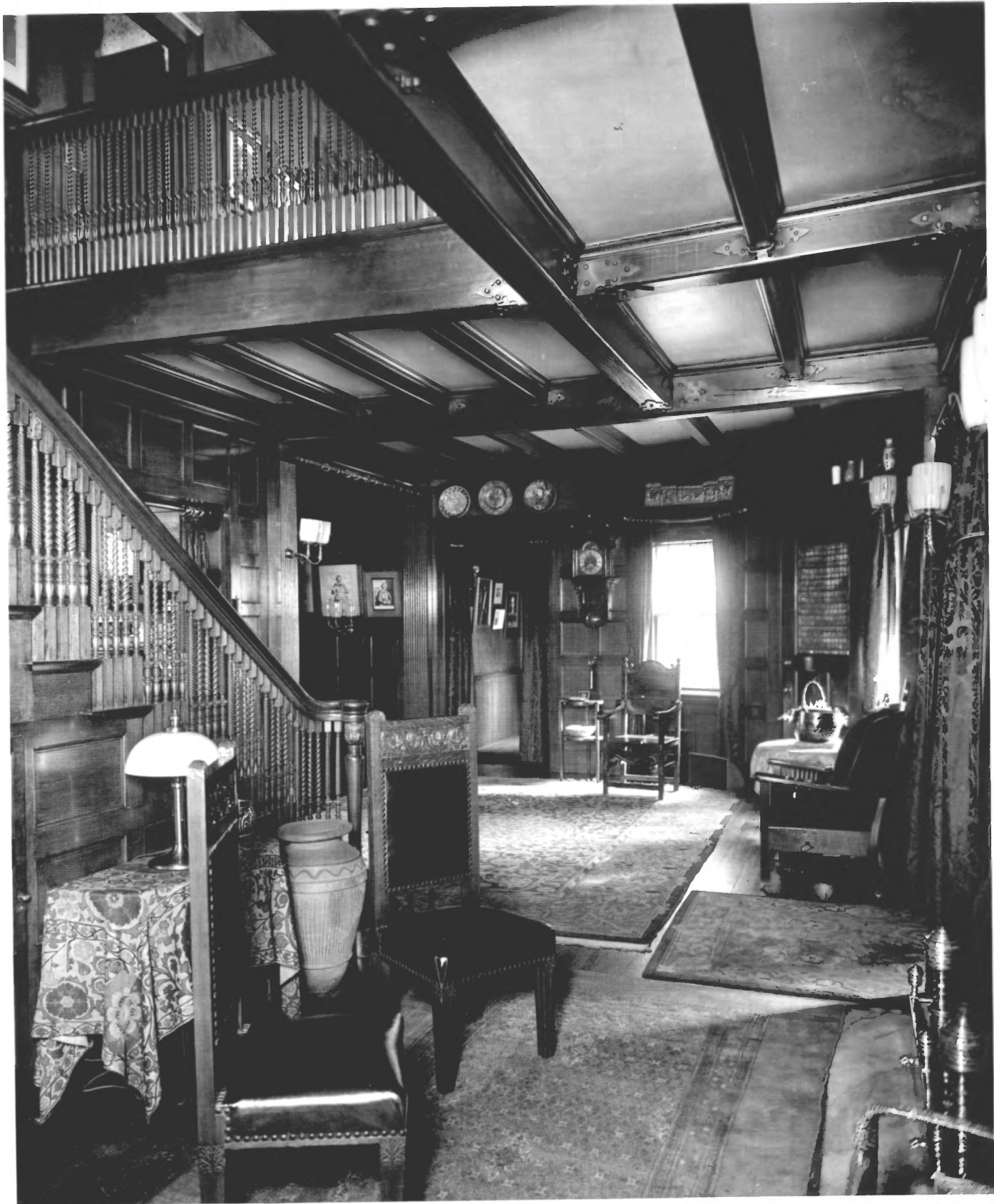
Glessner House, Chicago, Illinois Interior Stair hall, first floor (South)
